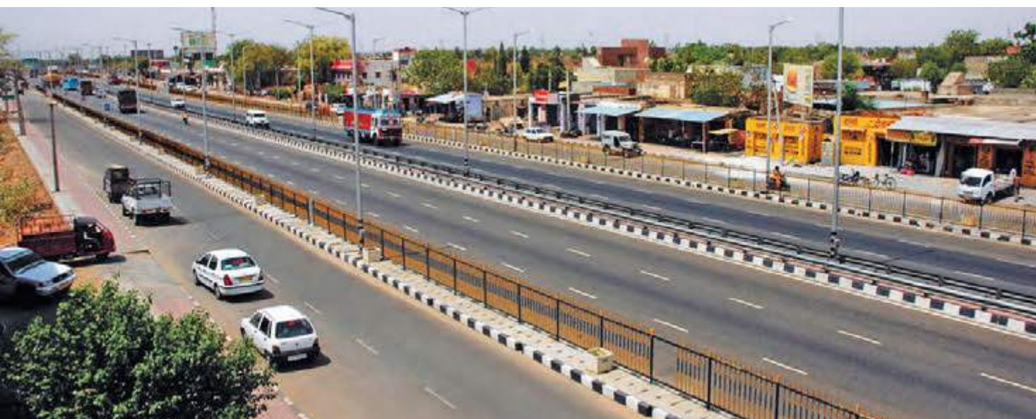
A two-lane road transformed into a 6-lane highway
