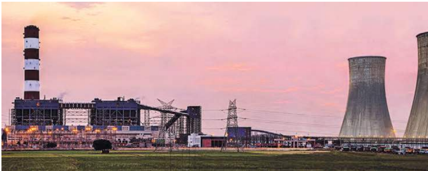
2 x 700 MW Rajpura Thermal Power Plant, Punjab
