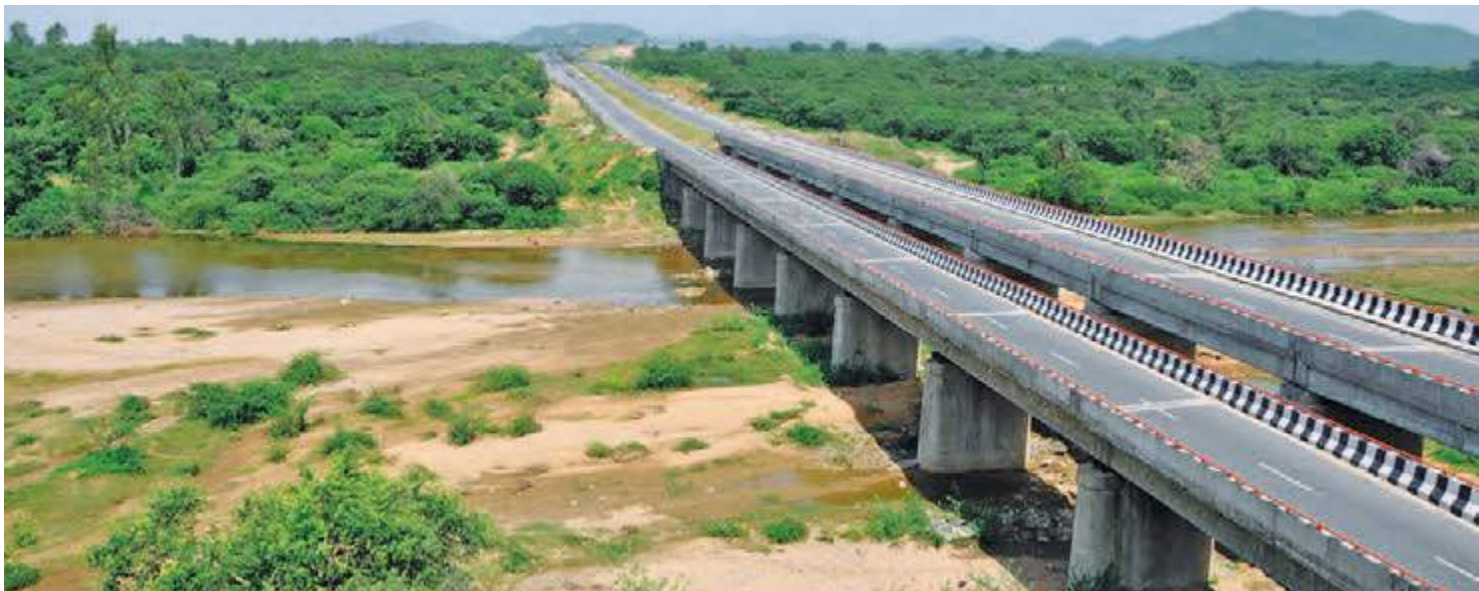
NH-14 Palanpur-Swaroopganj Highway
