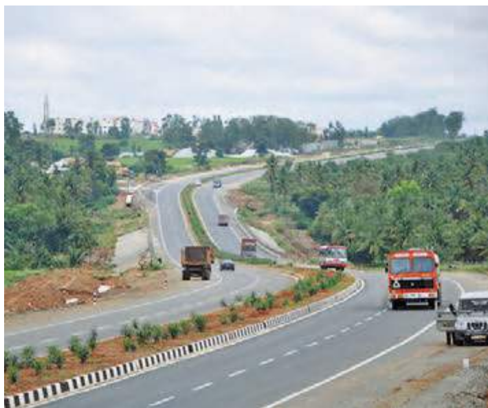
Devihalli Hassan Toll Road
