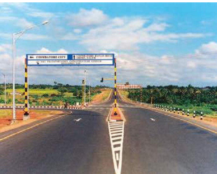
Coimbatore Bypass Road
