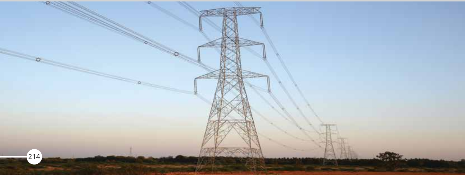
Kudgi Power Transmission Line project, Karnataka
