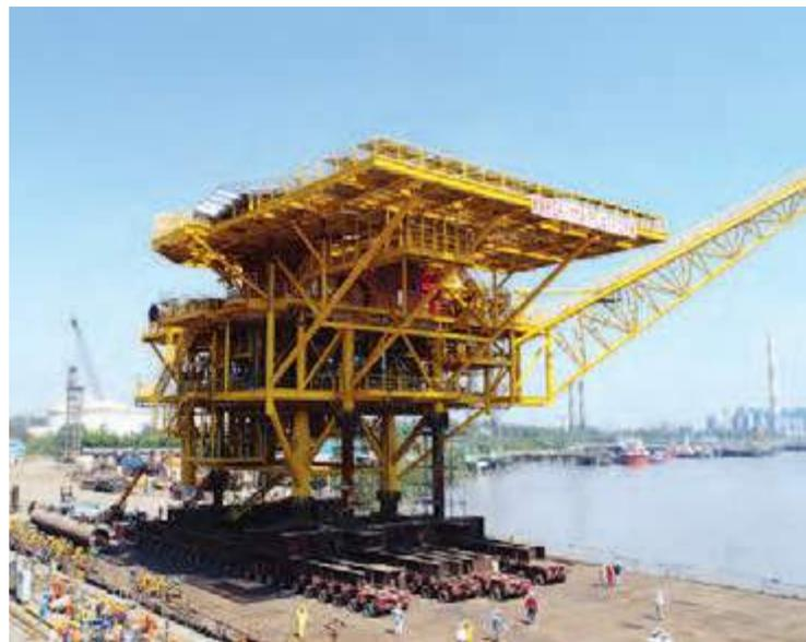
Load-out of BSE-11A Topside for Bassein Development 3 Well Platform & Pipeline Project of ONGC from Modular Fabrication Facility at Hazira, India
