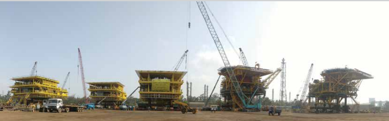
Production Deck Modules (PDMs) for Saudi Aramco ready for despatch from Modular Fabrication Facility, Hazira
