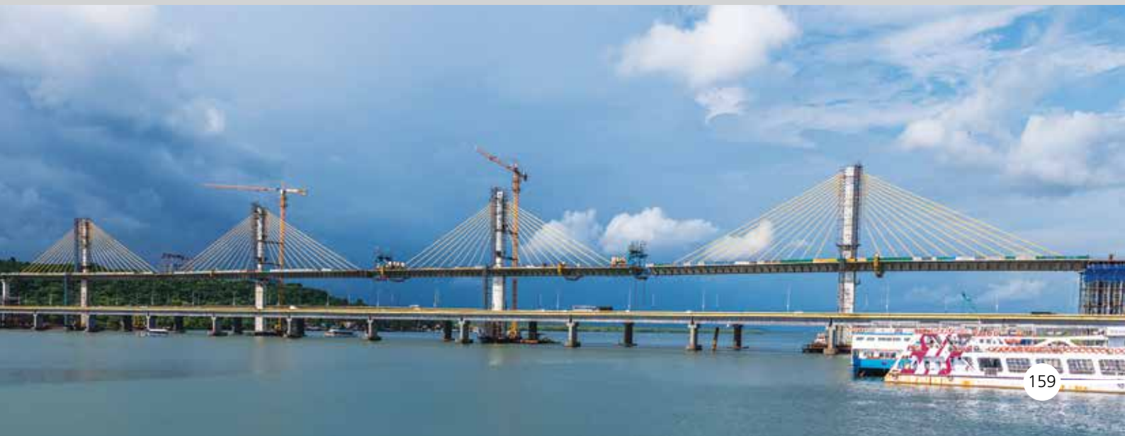
620 m long cable-stayed bridge across the river Mandovi in Panaji, Goa
