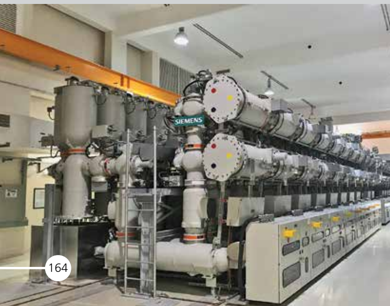
220 kV Gas Insulated Substation at Mehairja, Qatar
