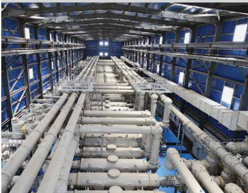
756 kV Gas Insulated Substation at Varanasi
