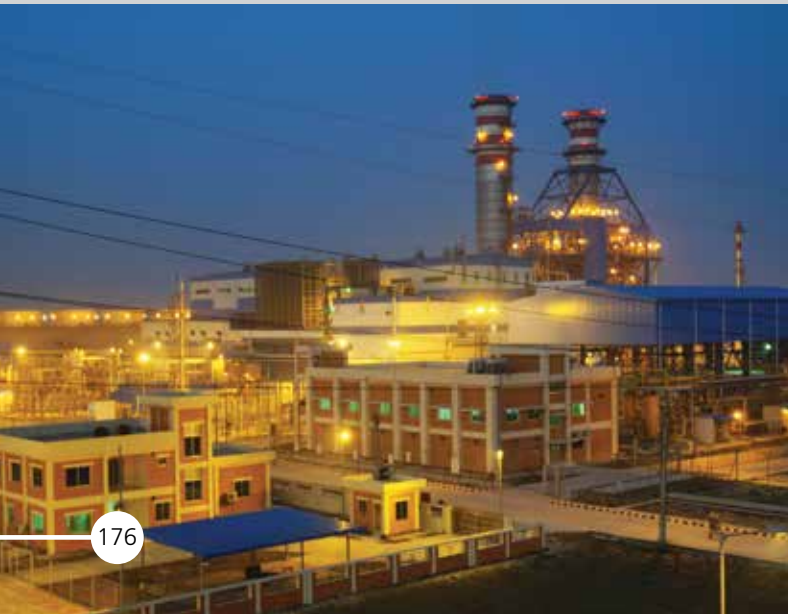
360 MW Combined Cycle Power Plant, Bheramara, Bangladesh, built on EPC basis
