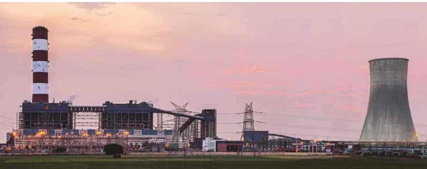
*Rajpura 2x700 MW Supercritical Technology based Thermal Power Plant*
