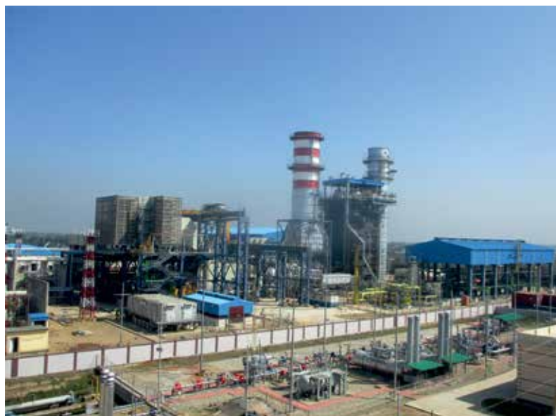
400 MW Combined Cycle Power Plant, Bibiyana-III, Bangladesh
