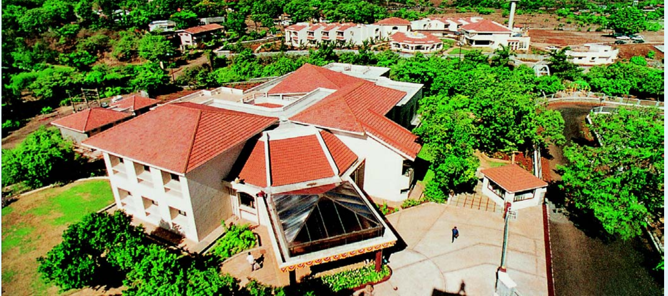
A temple of learning in a serene environment - L&T's Management Development Centre at Lonavala.
