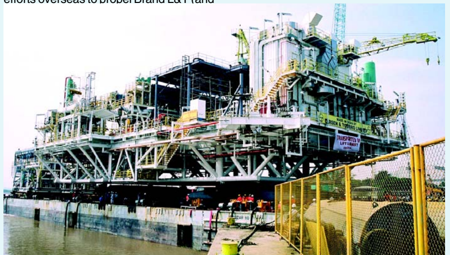
A giant process platform sails off from L&T's Hazira facility bound for the oil and gas fields of Abu Dhabi.
