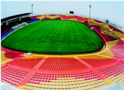
Qatar is slated to host the next Asian Games, and L&T assists in the preparation by building a sports stadium and the Games Village complex.
