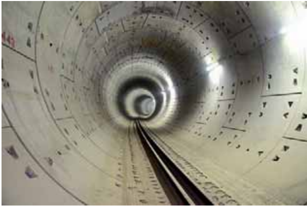
Tunnel for Delhi Metro. L&T has built underground and elevated corridors for the metro in major cities.
