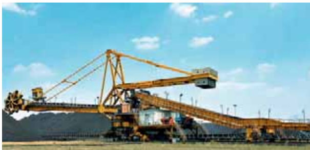
Coal-handling plant executed by L&T at Koderma in Jharkhand. L&T is a single-point solutions provider for a comprehensive range of material-handling systems.
