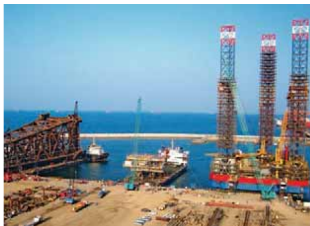
A jack-up rig along with a wellhead platform and a jacket at L&T's Modular Fabrication Yard in Sohar, Oman.
