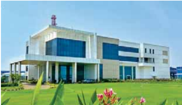
The Administrative Building at L&T's Kattupalli Campus has won 'LEED Platinum Certification' from the globally respected United States Green Building Council (USGBC)
