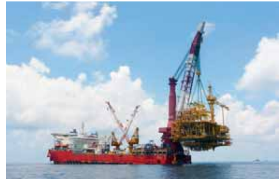
EPC services for the hydrocarbon sector include installation offshore
