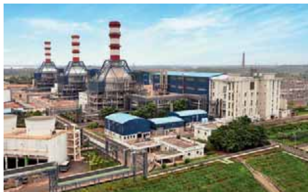
Natural gas-fired combined-cycle power plant built by L&T at Vemagiri in Andhra Pradesh.
