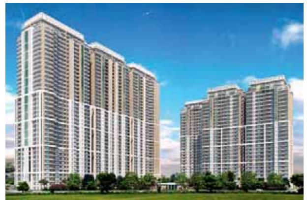
High-rise towers for a residential project in Delhi. The Buildings & Factories business provides world-class ‘Concept-to-Commissioning’ solutions across various building segments.
