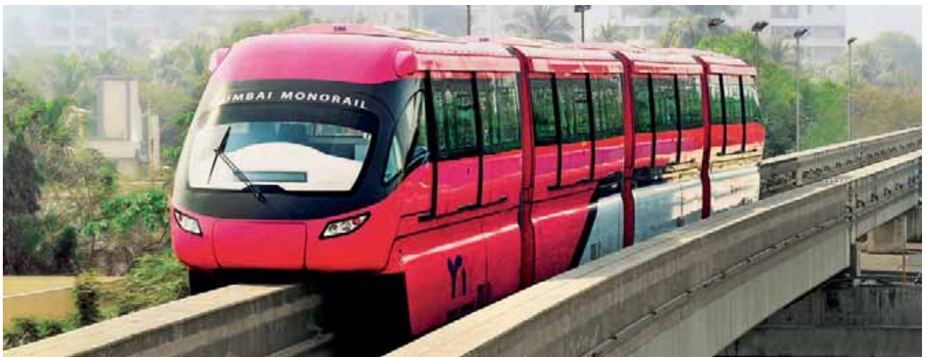
India's first monorail, in Mumbai, built and commissioned by L&T.
