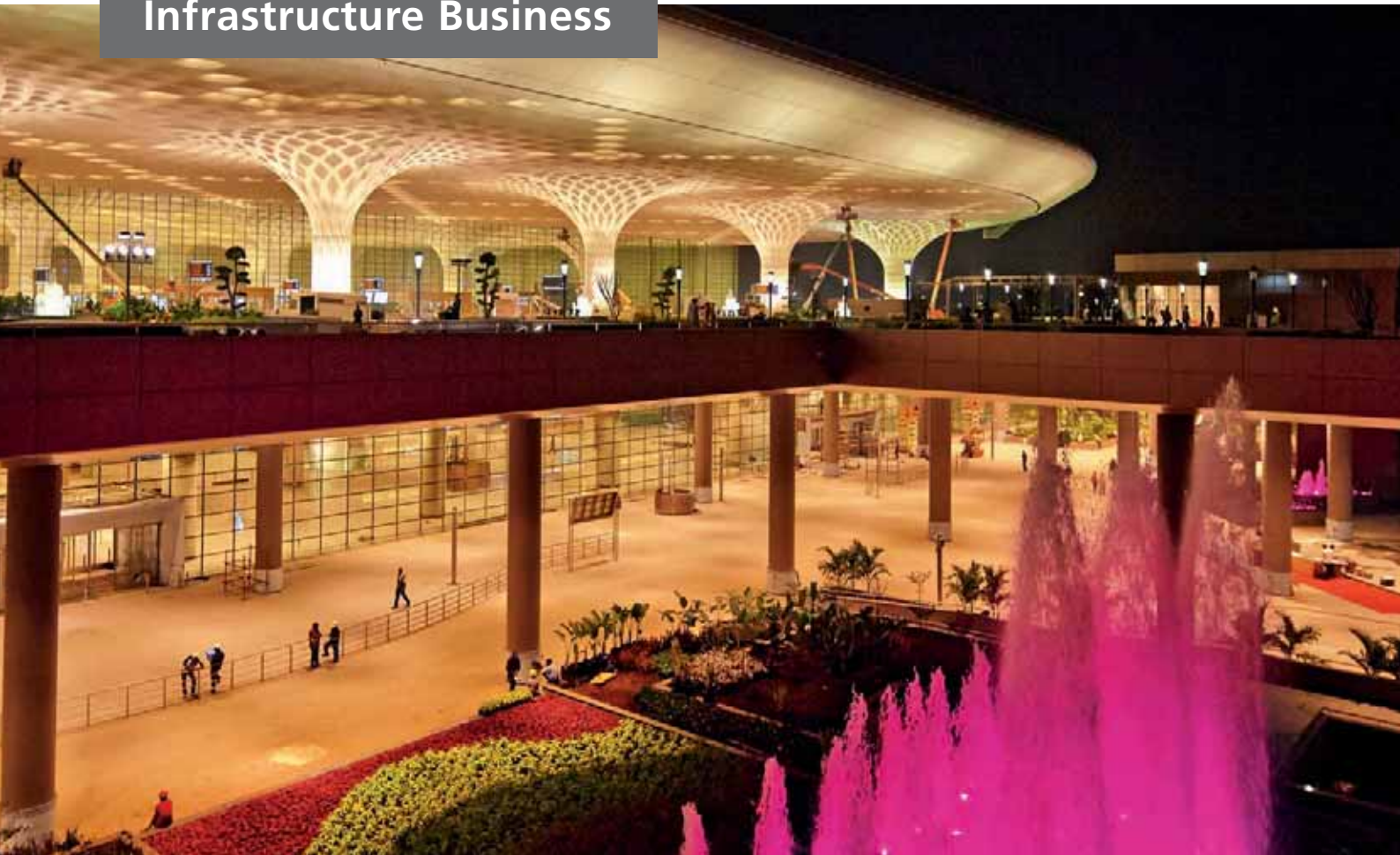
The new Gateway of India - Terminal 2 at Mumbai Airport. L&T has constructed several modern airports that include New Delhi, Bengaluru and Hyderabad in India. The Salalah International Airport in Oman is at an advanced stage of construction.
