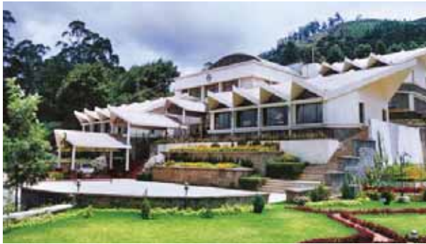
At L&T's Switchgear Training Centres around the country, the emphasis is not on 'selling' of brand or product, but on ensuring that customers adopt good electrical practices and gain the maximum value from switchgear.
