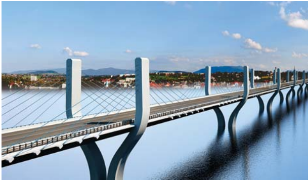
Perspective of the bridge over the Narmada, Gujarat - one of the longest of its kind to be built in India.
