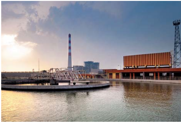
Water pre-treatment plant at Sagardighi, West Bengal
