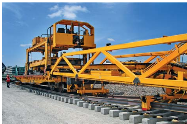
Automated track-laying machine deployed at the prestigious Dedicated Freight Corridor project.
