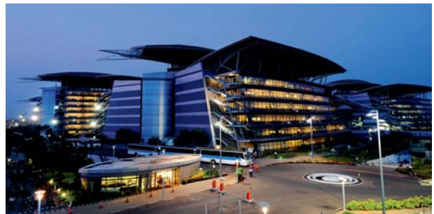
IT complex built by L&T for a software major. The high percentage of 'repeat orders' that L&T secures across all its businesses is possibly the most accurate reflection of customer confidence in the Company's offerings.
