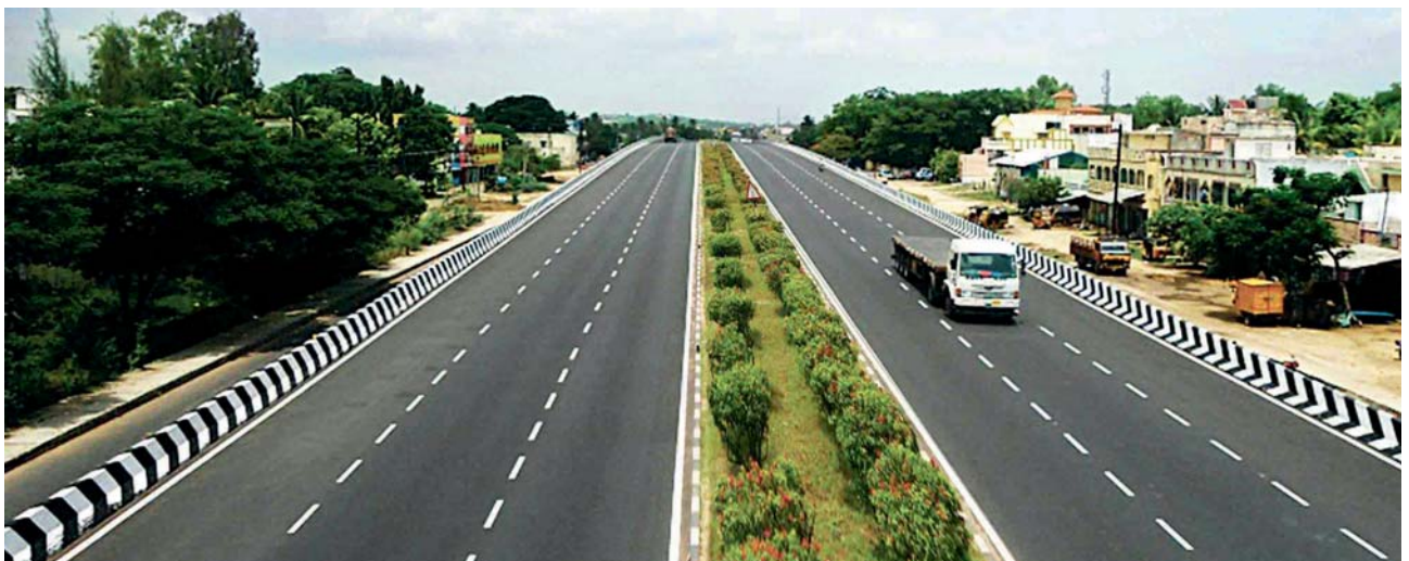
The six-lane, 148.34 kms stretch of road on NH-46 from Krishnagiri to Walajahpet in Tamil Nadu
