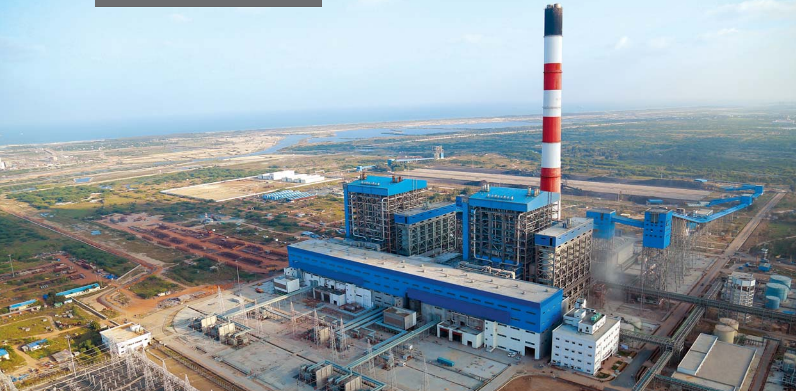
2x800 MW supercritical thermal power plant, Krishnapatnam, Andhra Pradesh. L&T provides EPC solutions for coal and gas-based power plants
