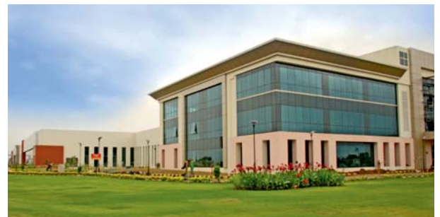
L&T's Switchgear Training Centre in Vadodara. At all L&T centres, the emphasis is not on 'selling' of brand or product, but on ensuring that customers adopt good electrical practices and gain the maximum value from switchgear.
