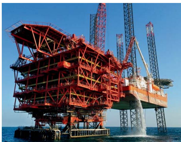
Wellhead platform commissioned off the coast of Abu Dhabi
