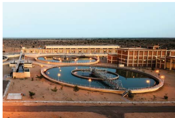
172 MLD Lift Water Supply Project, Rajasthan. L&T has designed and constructed numerous water reservoirs, pipelines and distribution systems.
