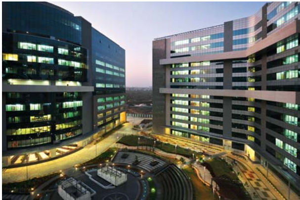
L&T has built over 150 IT parks and commercial complexes in India and neighbouring countries.
