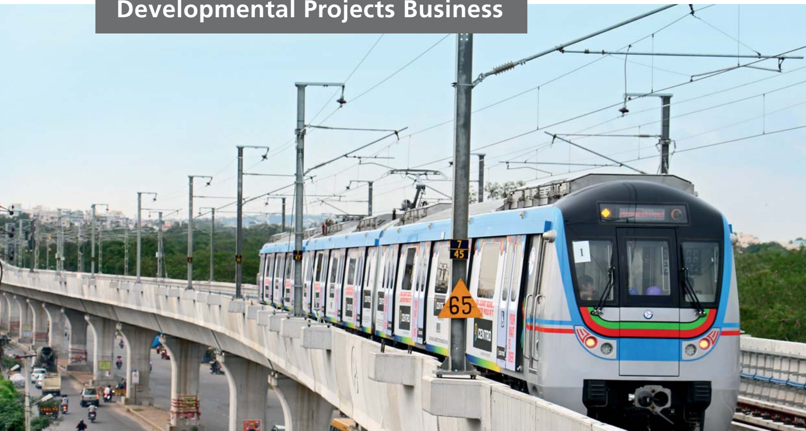
The Hyderabad Metro Rail Project - the world's largest Public-Private-Partnership (PPP) project in the metro sector
