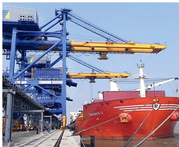
Unloading operations on a Cape size vessel berthed at Dhamra Port, Odisha
