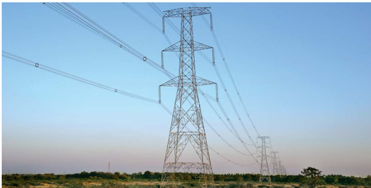
Kudgi Power Transmission Line project, Karnataka
