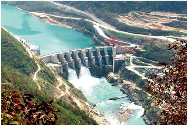
Hydroelectric power plant at the foothills of the Himalayas
