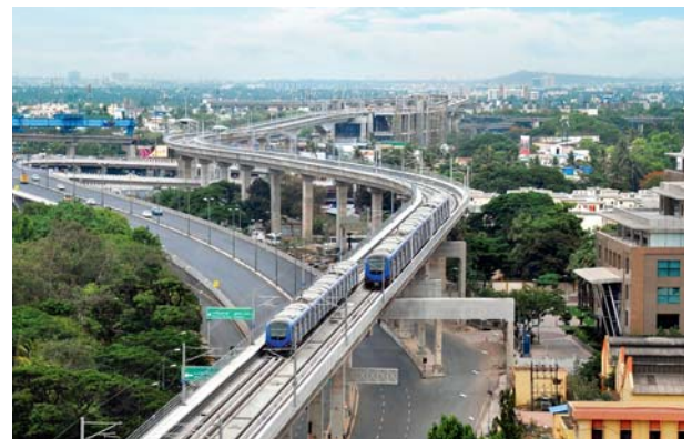
L&T is constructing the elevated and underground sections of the Chennai Metro and is involved in the Kochi and Lucknow Metro projects.
