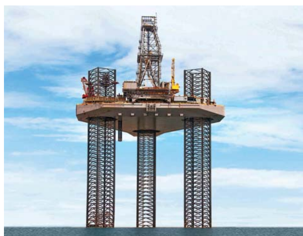
Major repair and upgradation was carried out on a jack-up rig
