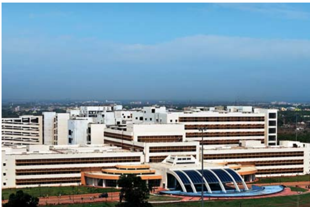
All India Institute of Medical Sciences Hospital, Bhubaneswar - one of the many healthcare institutions built by L&T in India and the Gulf.
