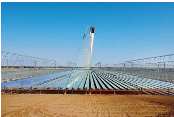
Asia's largest (125 MWe) solar thermal power plant in Rajasthan, based on high efficiency, CSP technology. L&T is the country's largest player in the field of solar plant construction.
