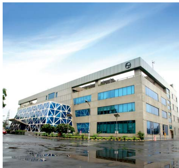
Sustainability begins at home. 'Unnati' - L&T's new facility in Navi Mumbai has achieved LEED (Leadership in Energy and Environmental Design) Gold Certification.
