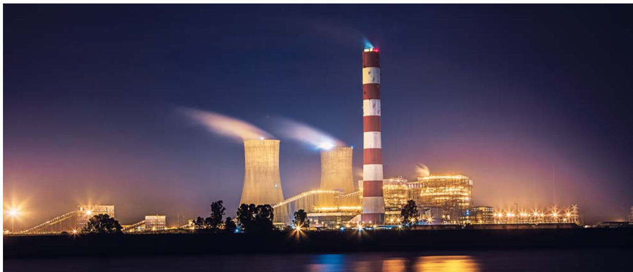
2x700 MW supercritical thermal power plant, Rajpura, Punjab. L&T provides EPC solutions for thermal power projects
