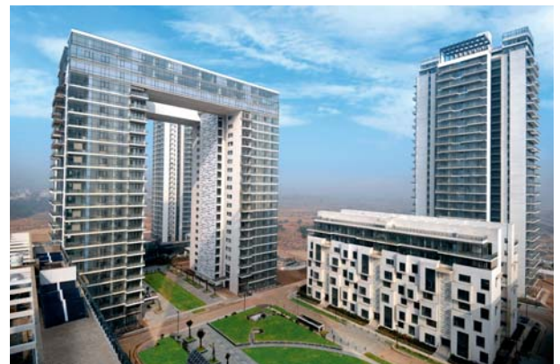
L&T is helping cities soar skywards by building a wide range of residential projects, from elite towers to mass-housing complexes.
