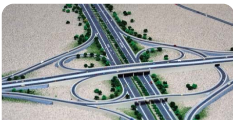
Sheikh Khalifa Interchange, UAE
