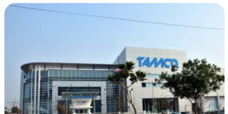
MV Switchgear Factory, Malaysia
