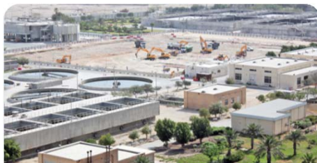
Water Treatment Plant, Doha
