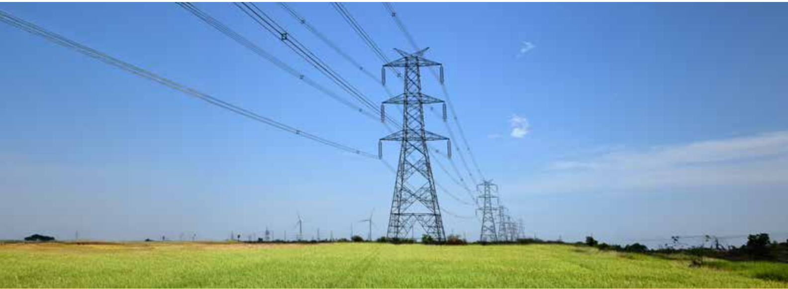
400kV Ottapidaram, Tamil Nadu
