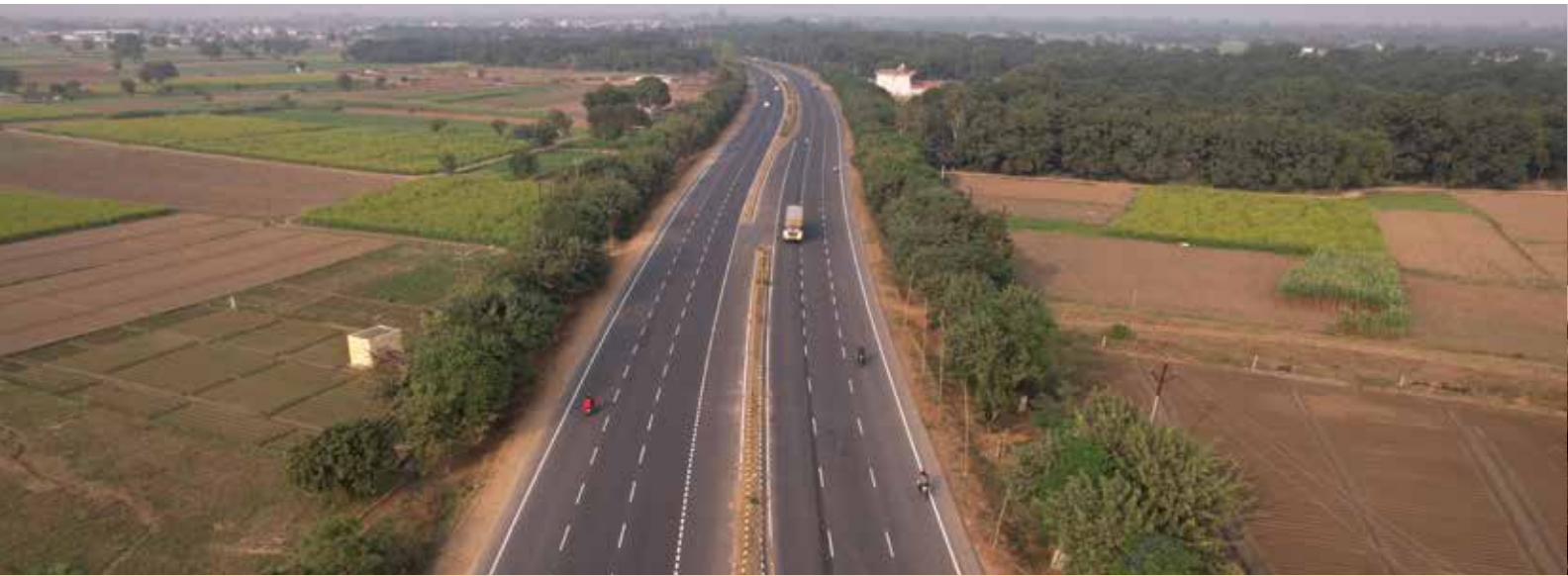
Meerut Aligarh Ghaziabad Road Project, Uttar Pradesh
