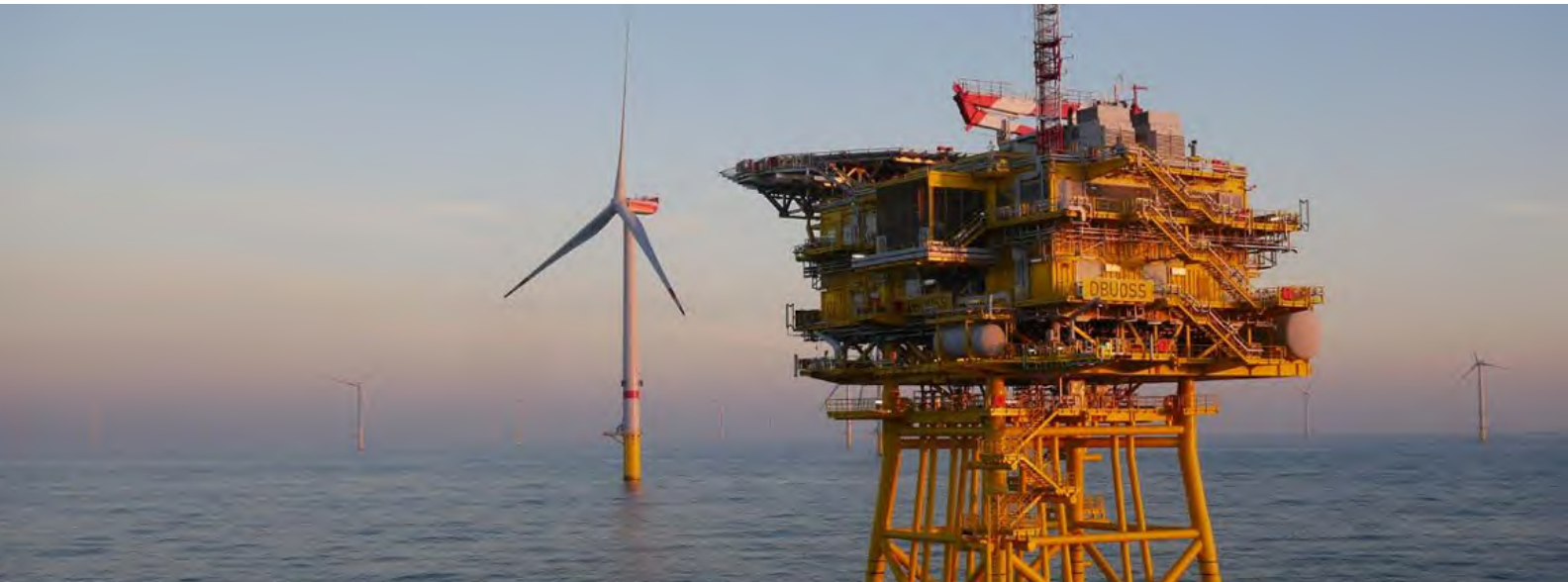
HVAC Offshore Substation
