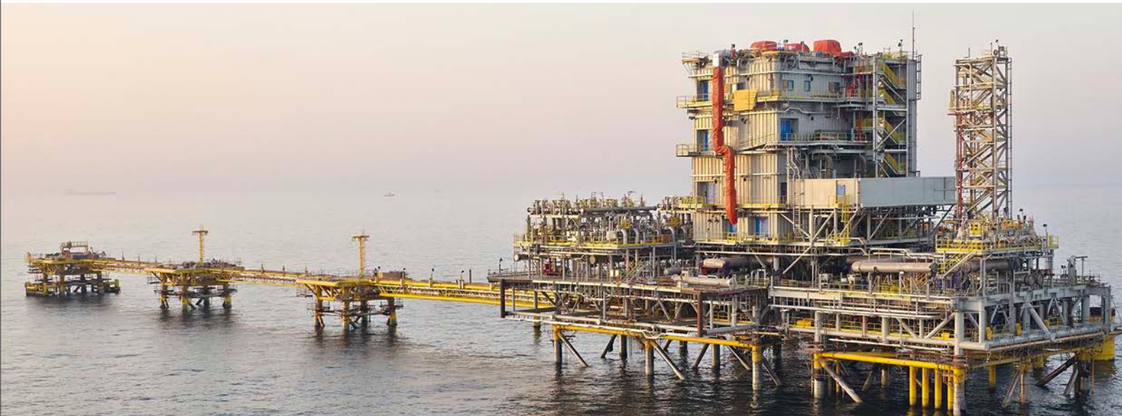
Marine Terminal Expansion Project, Juaymah NGL facilities, Kingdom of Saudi Arabia
