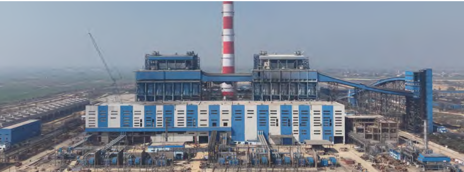
2x660 MW Buxar Thermal Power Plant, Bihar
