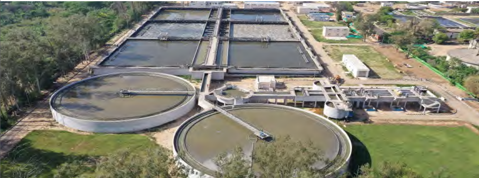
136 MLD Sewage Treatment Plant, Diggian, Chandigarh
