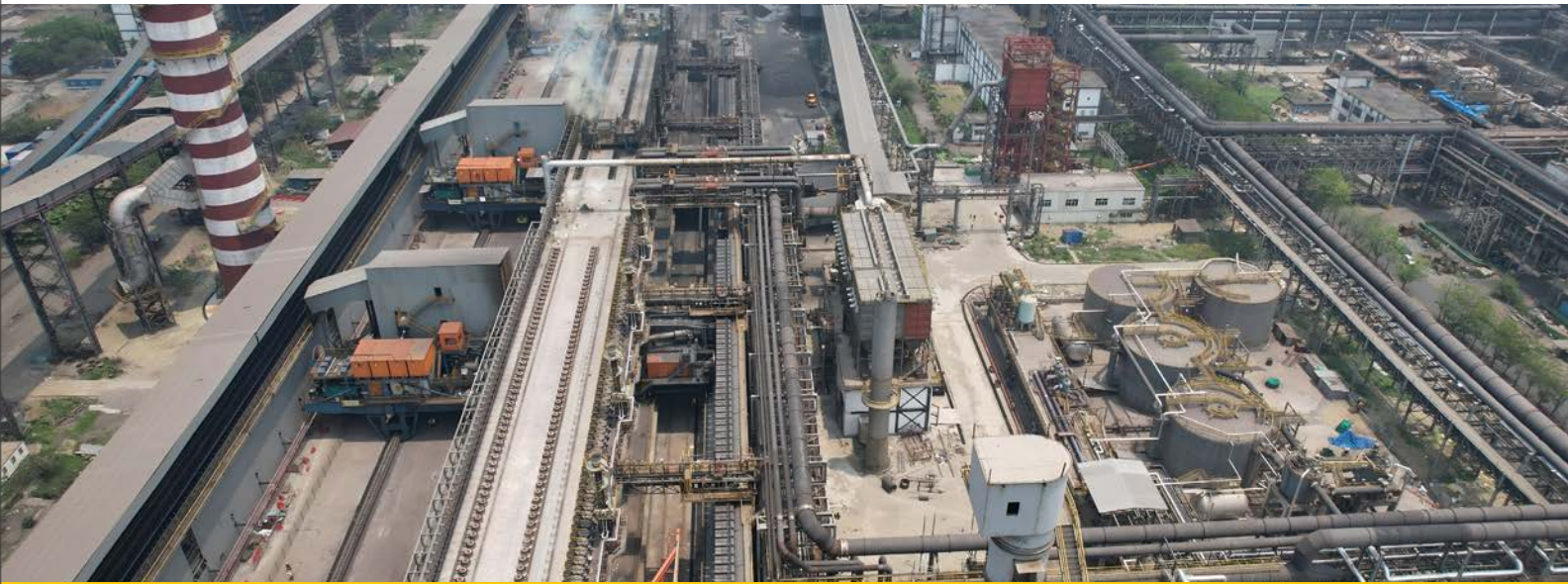
Kalinganagar Coke Oven Battery Project, Odisha
