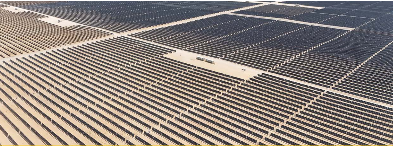
1.4 GW Al Kahfah Solar PV Project, Kingdom of Saudi Arabia
