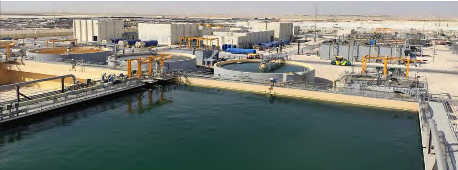
10 MLD Integrated Industrial Effluent Treatment Plant, Qatar
