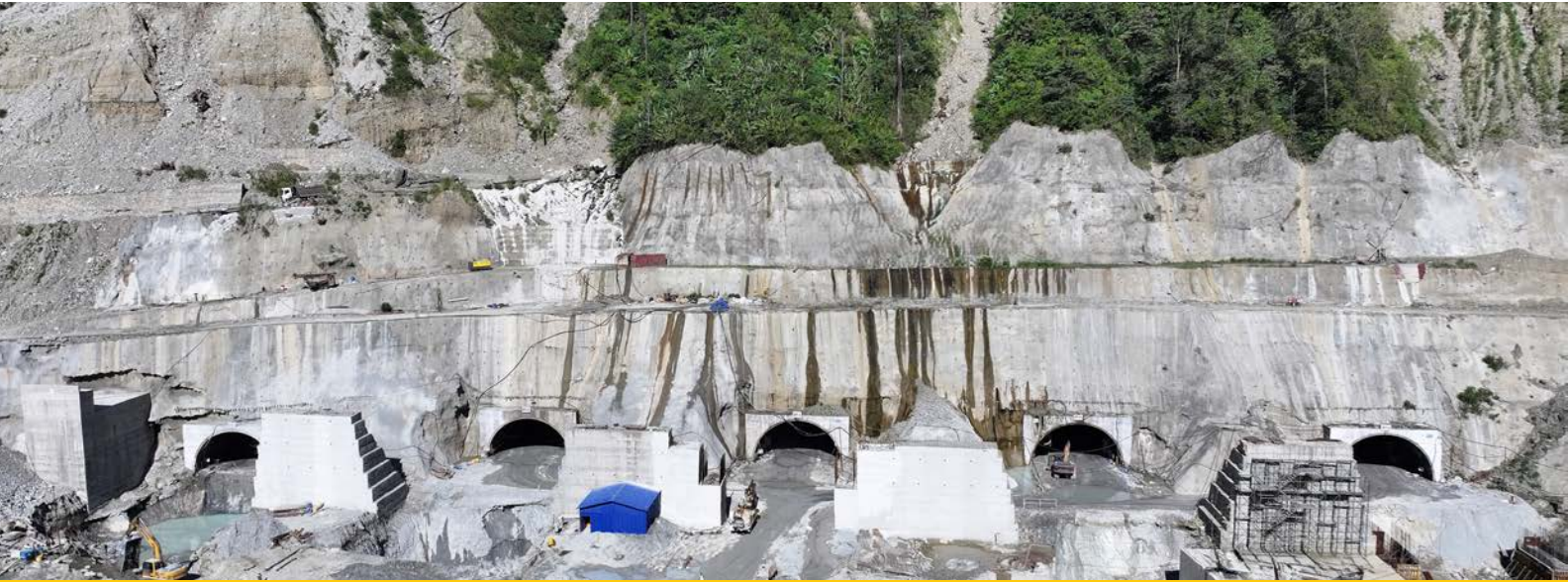
Dibang Multipurpose Project Lot-2, Diversion Tunnel Portal, Arunachal Pradesh
