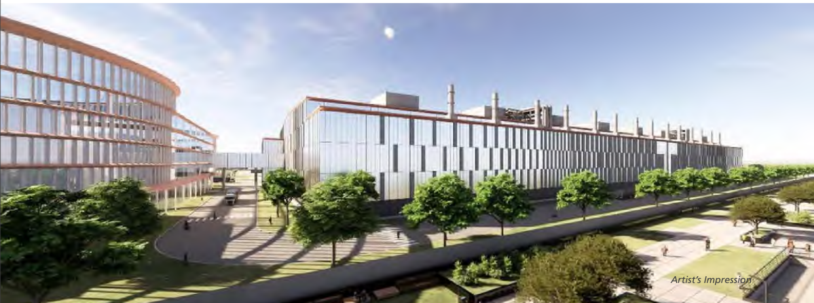
Semiconductor FAB Plant, Dholera, Gujarat
