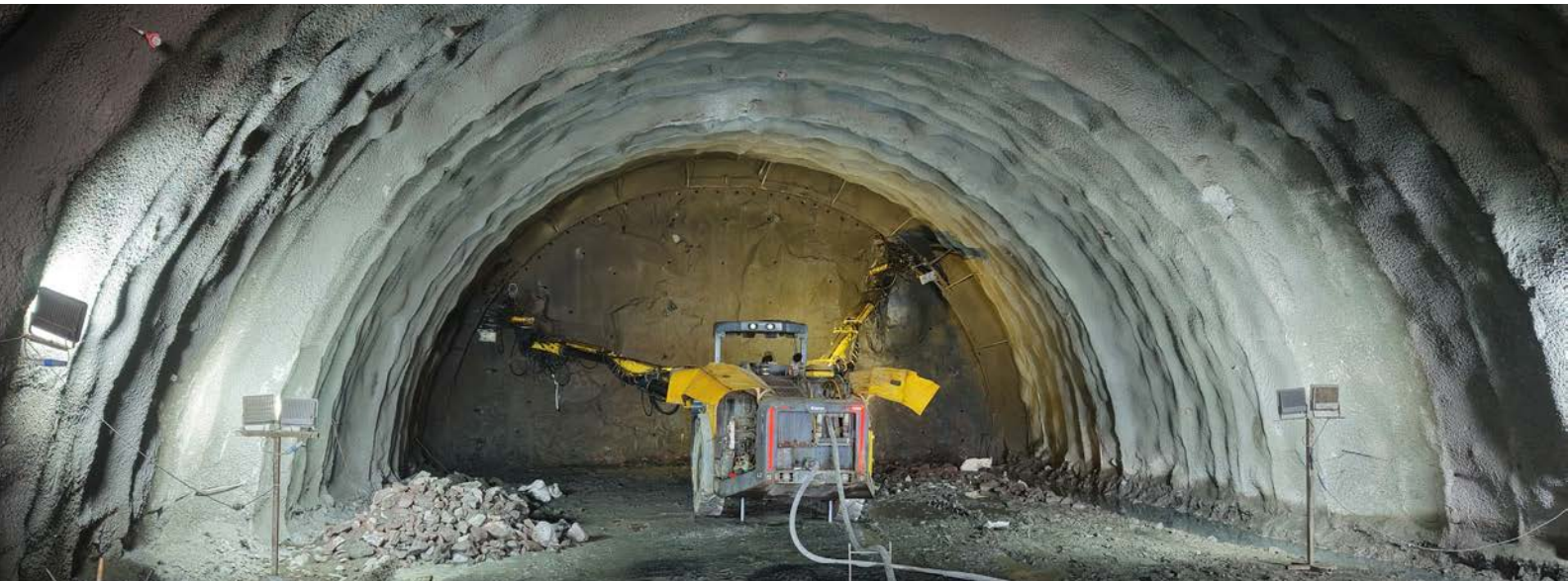
NATM tunnel MT05 of length 1,480 Rmt, Mumbai-Ahmedabad High-Speed Rail Package C3, Palghar, Maharashtra
