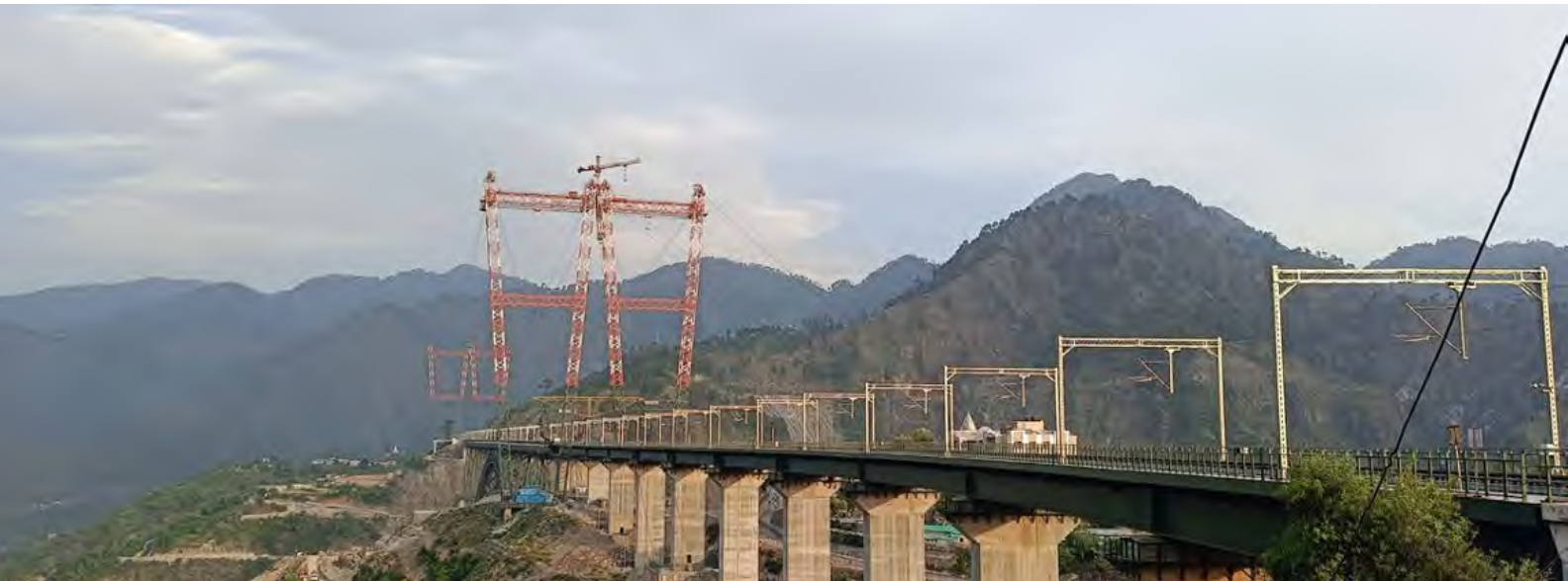
Electrification in Katra-Dharam section of USBRL including Chenab and Anji Khad bridges using Flexible and Rigid OCS, Jammu & Kashmir
