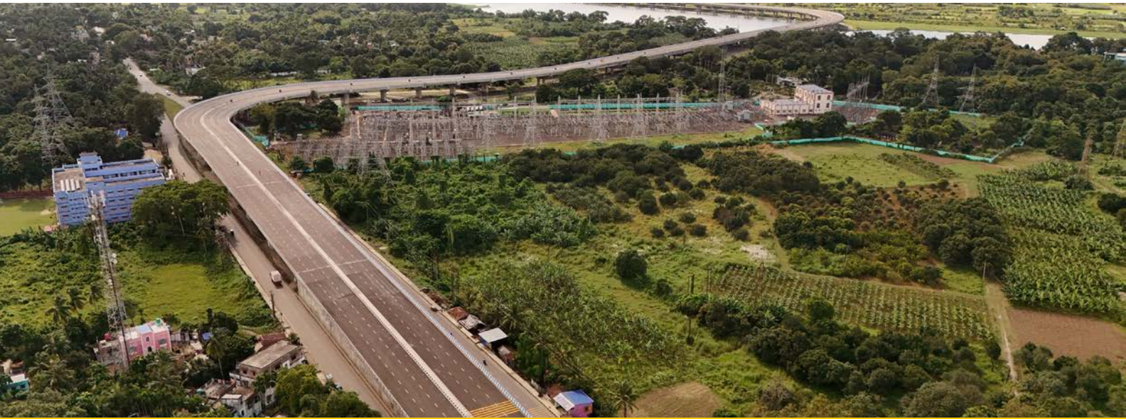
Second Iswar Gupta Setu project, extradosed bridge over the Hooghly River connecting Kalyani and Bansberia in West Bengal
