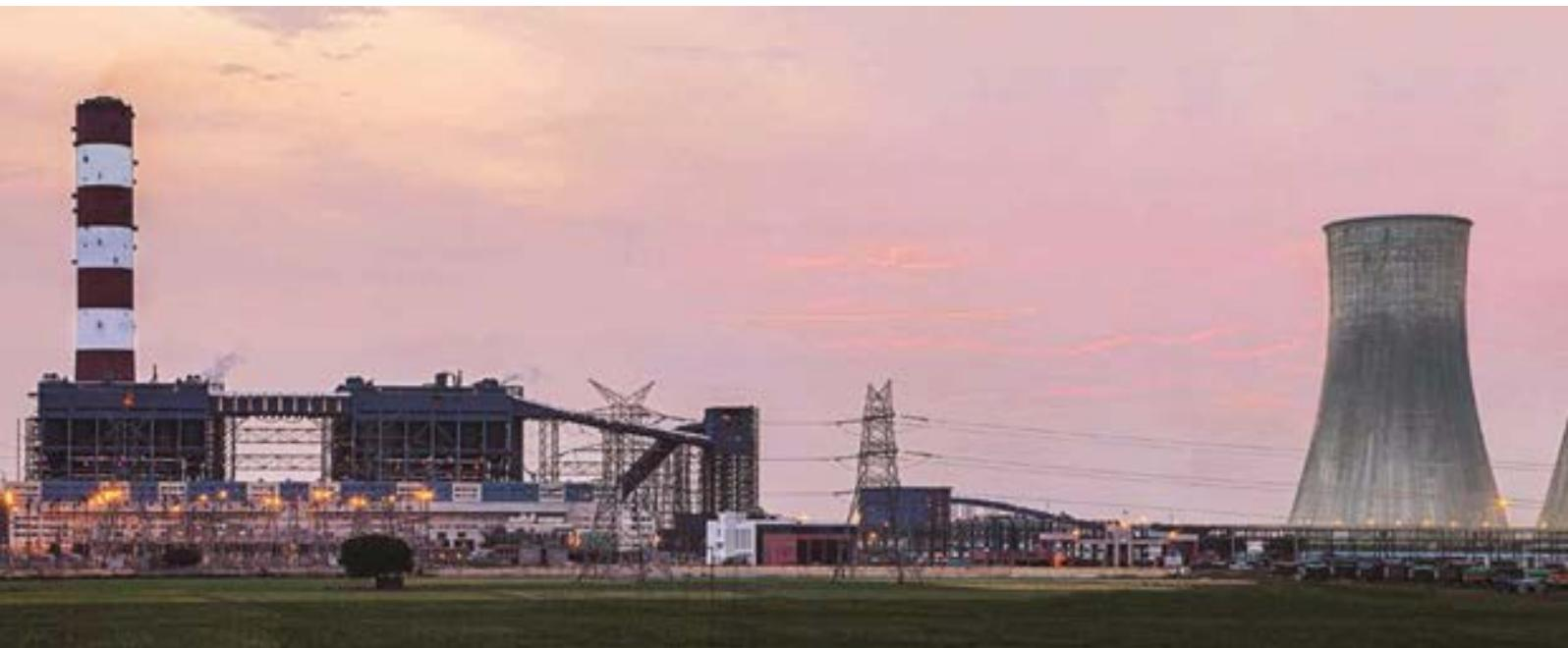
2x700 MW Supercritical Technology based Thermal Power Plant at Rajpura
