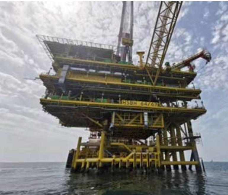
One of three gas PDMs installed in Hasbah and Arabia Offshore, Saudi Arabia
