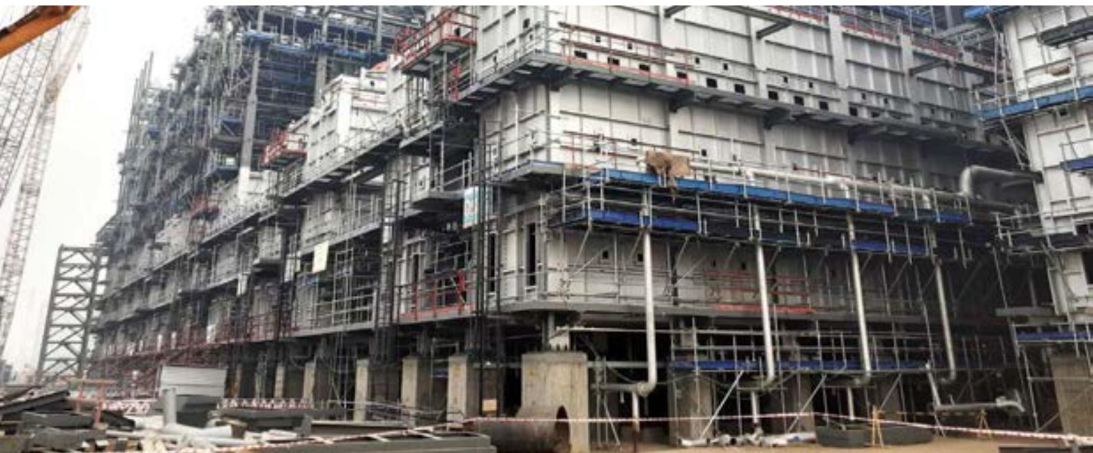
Convection modules built at MFF Hazira for HMEL Cracker Furnaces Project
