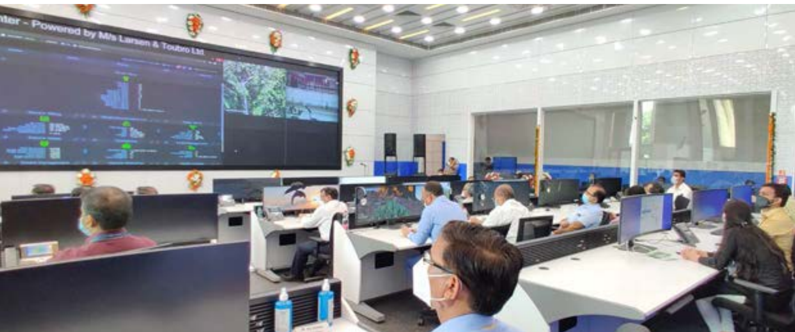
Integrated Command Control Centre for NDMC
