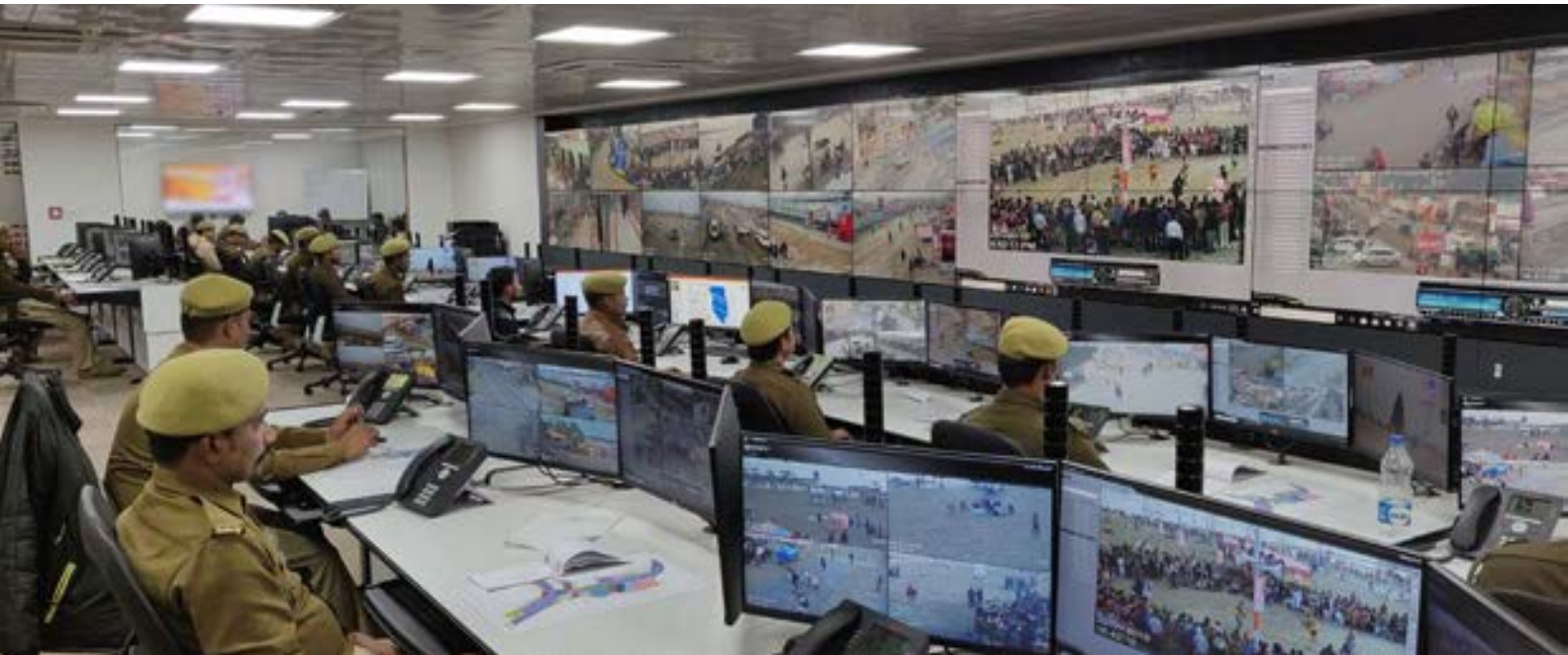
Command & Control Centre, Prayagraj
