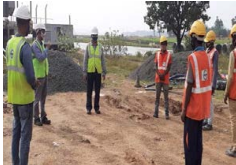
Workmen training helps enhance safety and productivity
