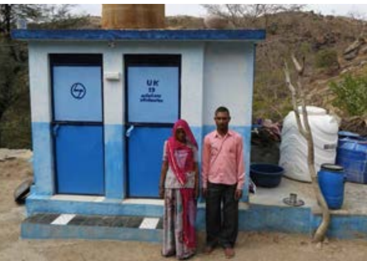
Toilet facilities were constructed to enable villages become open-defecation-free
