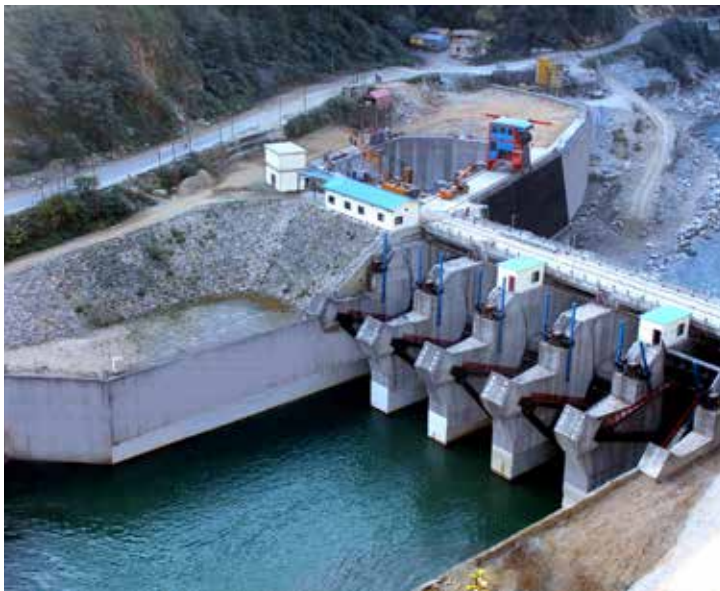
Singoli Bhatwari Hydro Power Project, Uttarakhand
