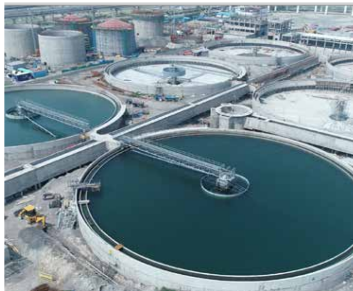
Secondary clarifiers under construction for 318 MLD Waste Water Treatment Plant, Coronation Pillar, New Delhi
