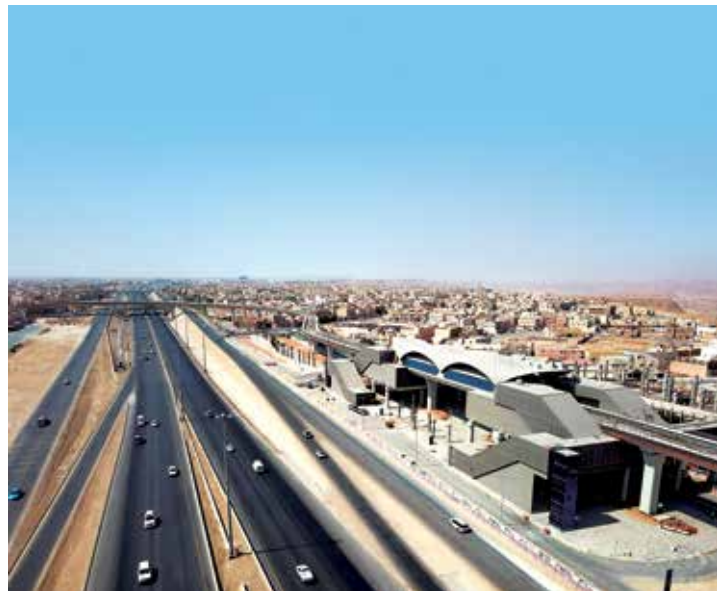
Riyadh Metro Line 3, Kingdom of Saudi Arabia
