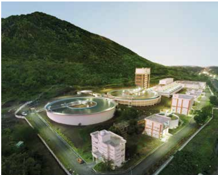
137 MLD Water Treatment Plant, Nashik, Maharashtra
