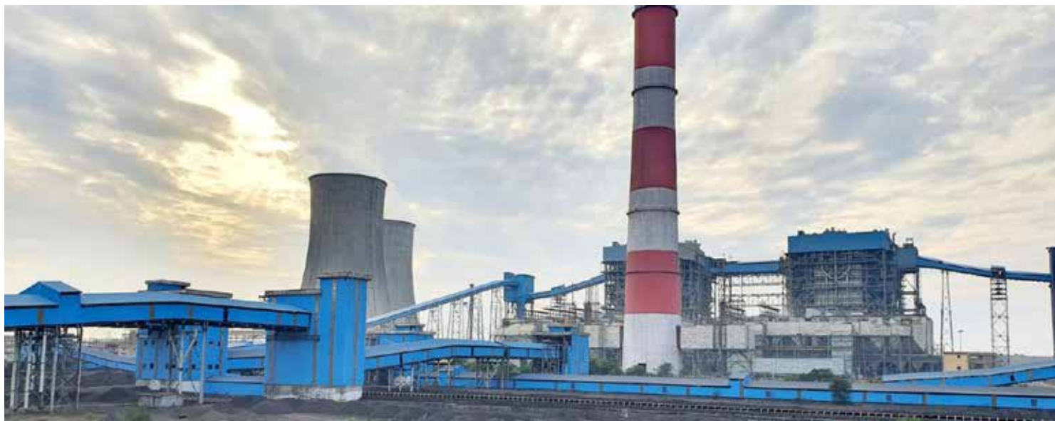
Chhabra Coal Handling Plant, Rajasthan
