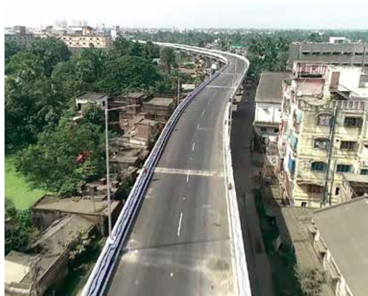
Bata Nagar Flyover, Kolkata, West Bengal
