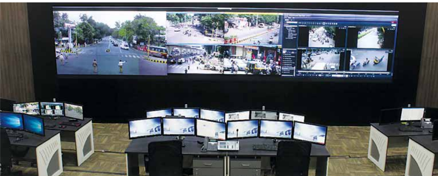
City Operation Centre, Nagpur
