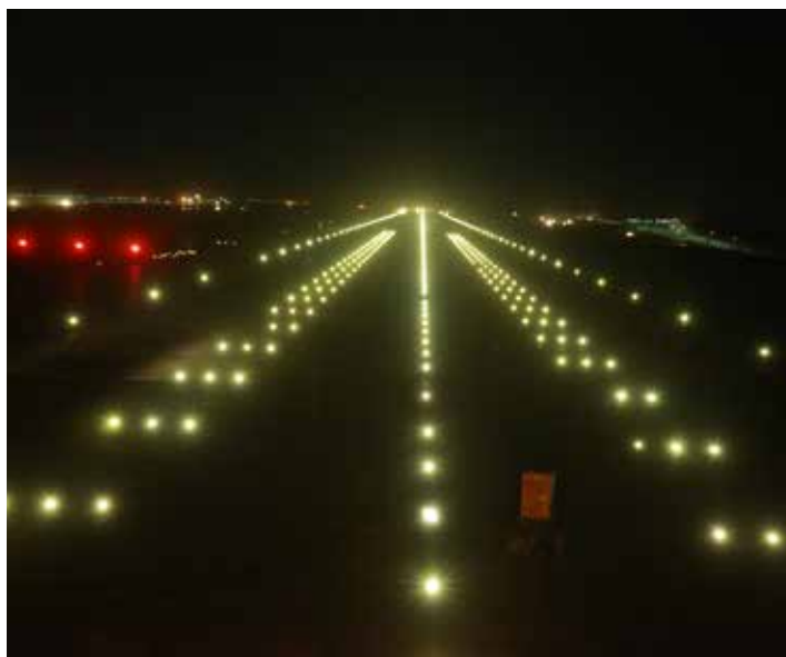
Runway for Bengaluru International Airport
