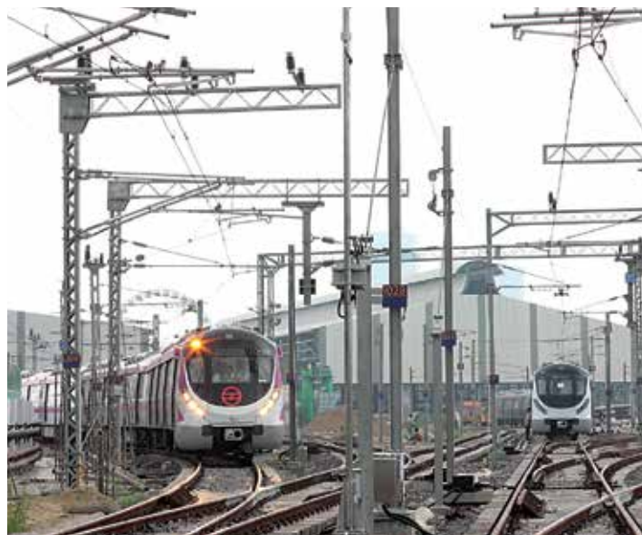
Overhead Electrification for Delhi Metro Phase 3
