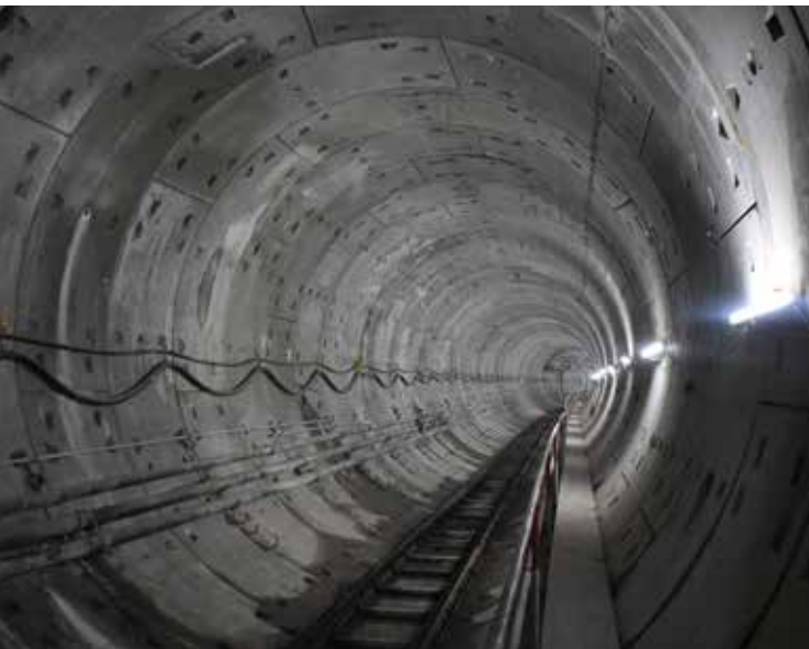
One of the underground tunnels for Mumbai Metro
