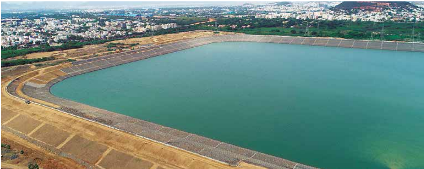
12 Million cu.m storage reservoir for Vizag Steel Plant, Andhra Pradesh
