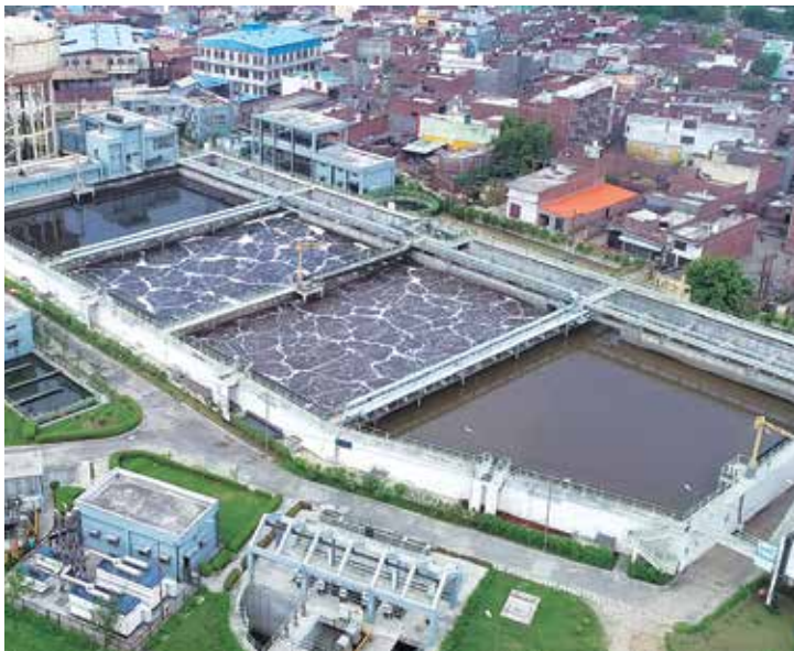
Moradabad Sewerage Treatment Plant, Uttar Pradesh
