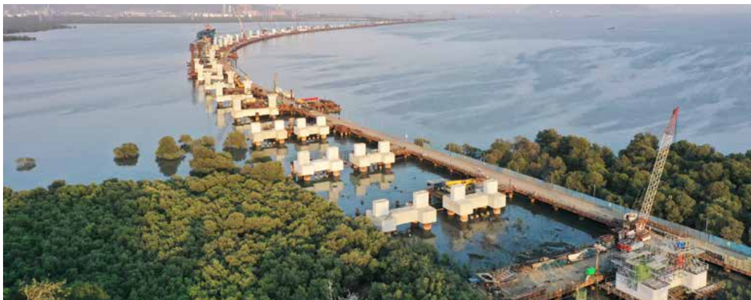
The Mumbai Trans Harbour Link
