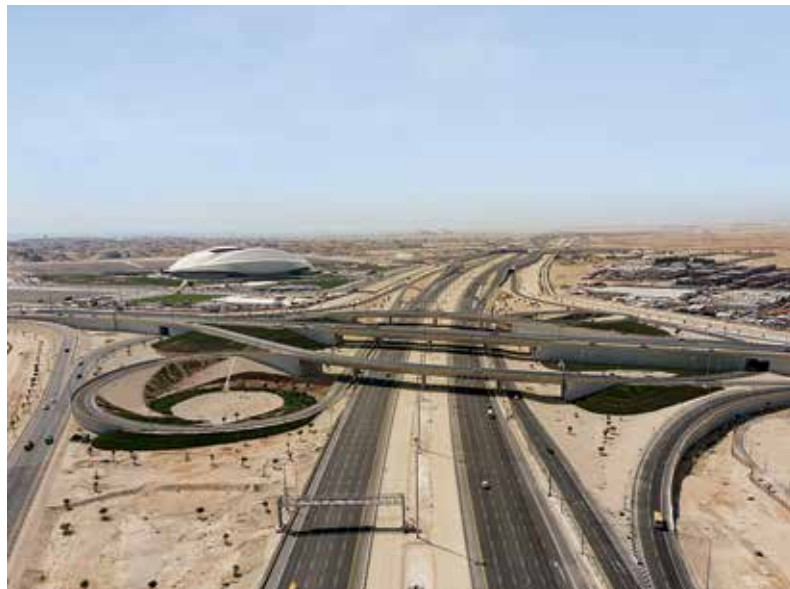
Al Wakrah Bypass Road Project, Qatar
