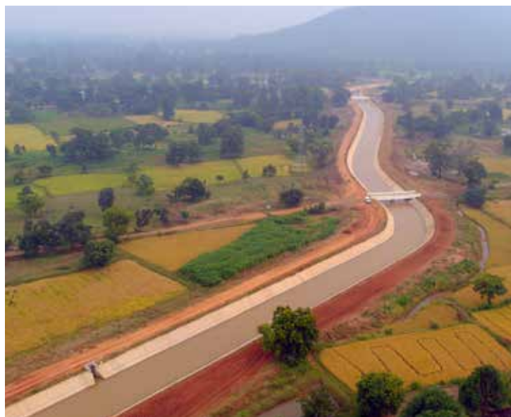
Lift Canal System for Upper Indravati Irrigation Project, Odisha
