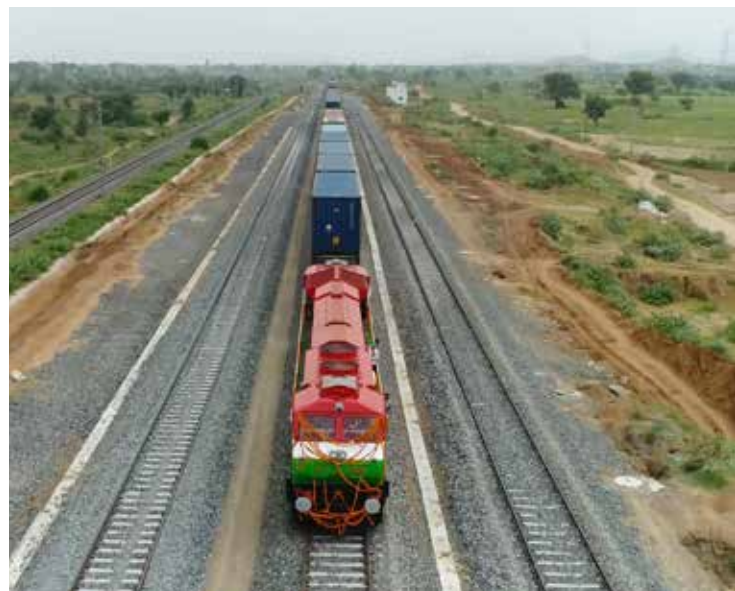
Trial run at Western Dedicated Freight Corridor
