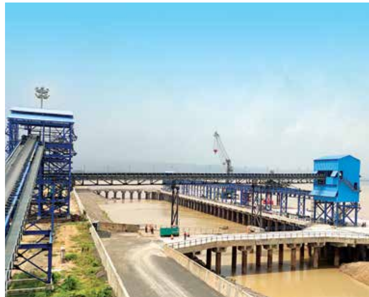
Multi-modal terminal at Sahibganj, Jharkhand
