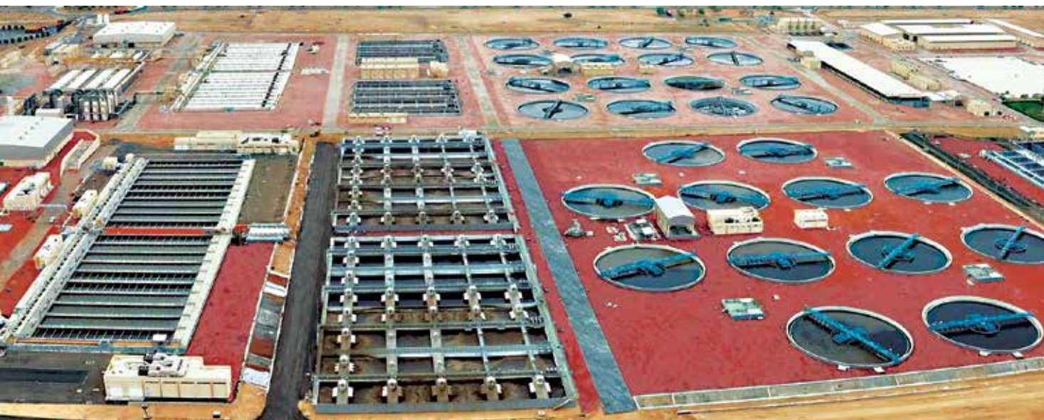
375 MLD Sewage Treatment Plant, Jebel Ali, UAE
