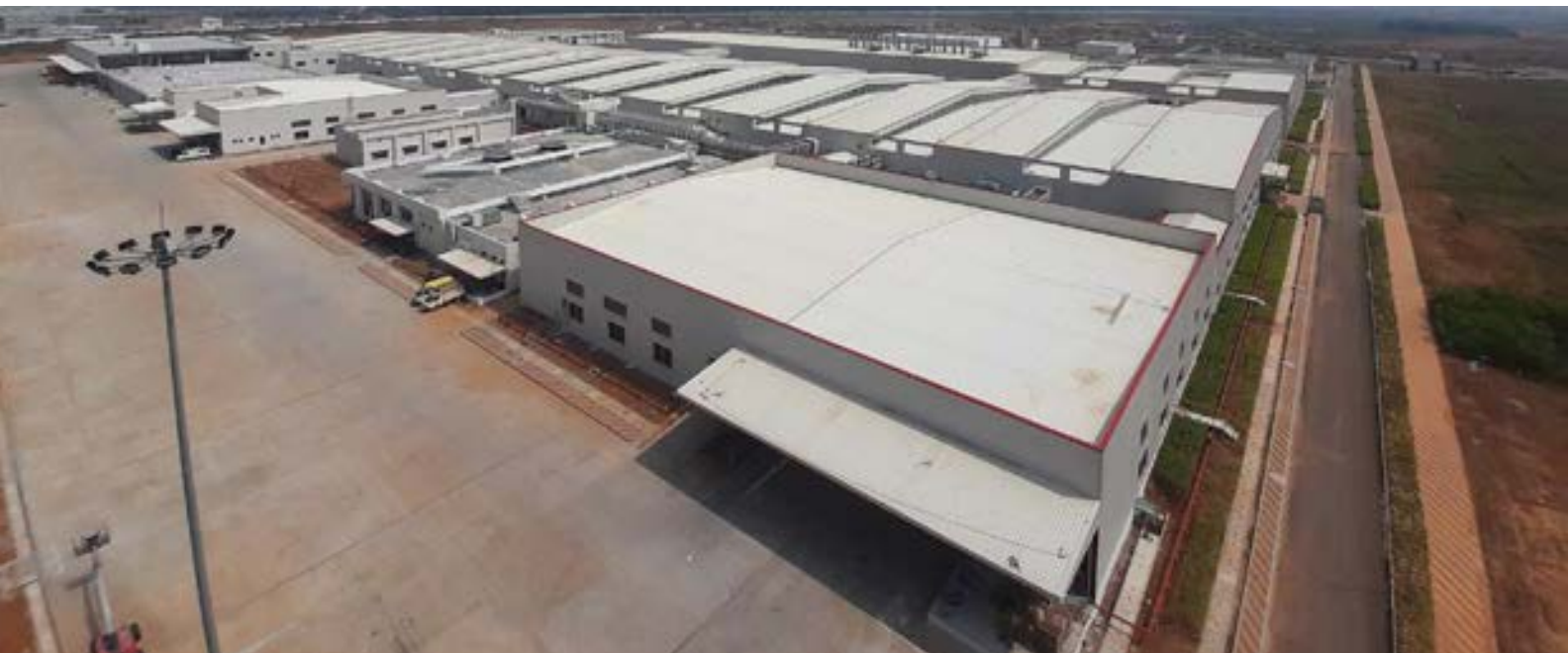
Hero Factory, Chittoor, Andhra Pradesh
