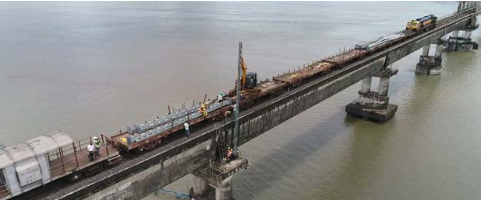
Roha-Verna Konkan Railway Electrification Project
