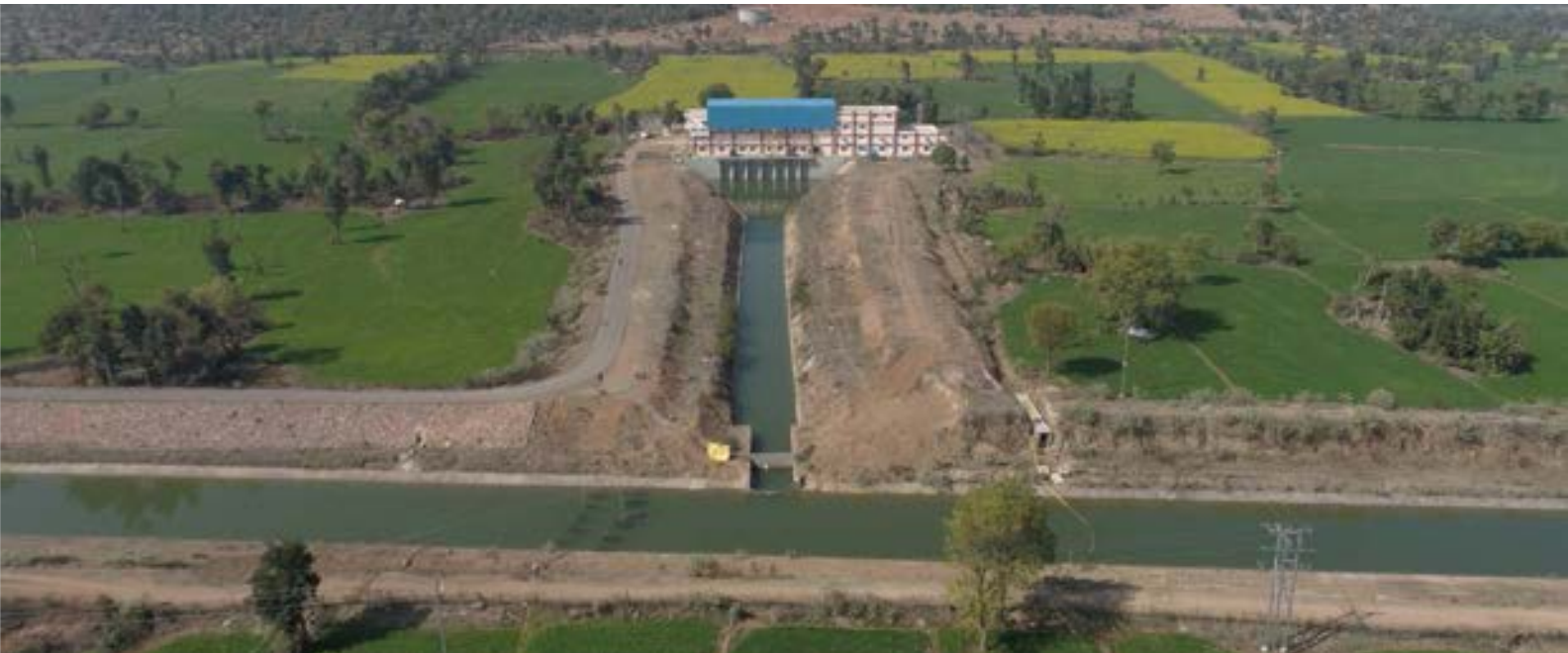
Bansujara Irrigation Scheme, Madhya Pradesh
