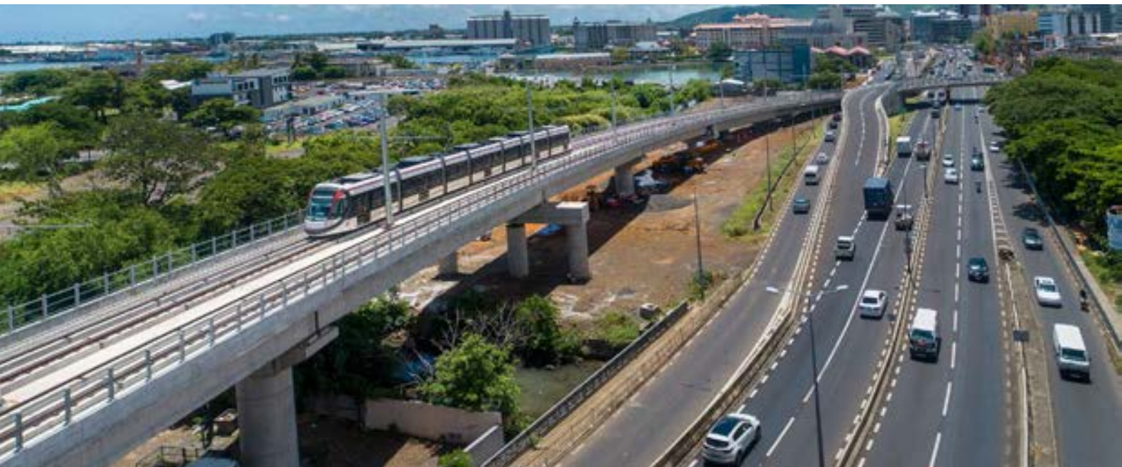
A section of the 13-km Phase 1 of the Mauritius Metro project
