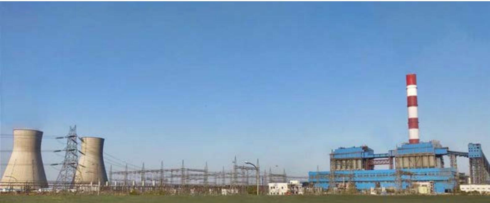
2x660 MW Shree Singaji Thermal Power Plant (Stage-II), Madhya Pradesh
