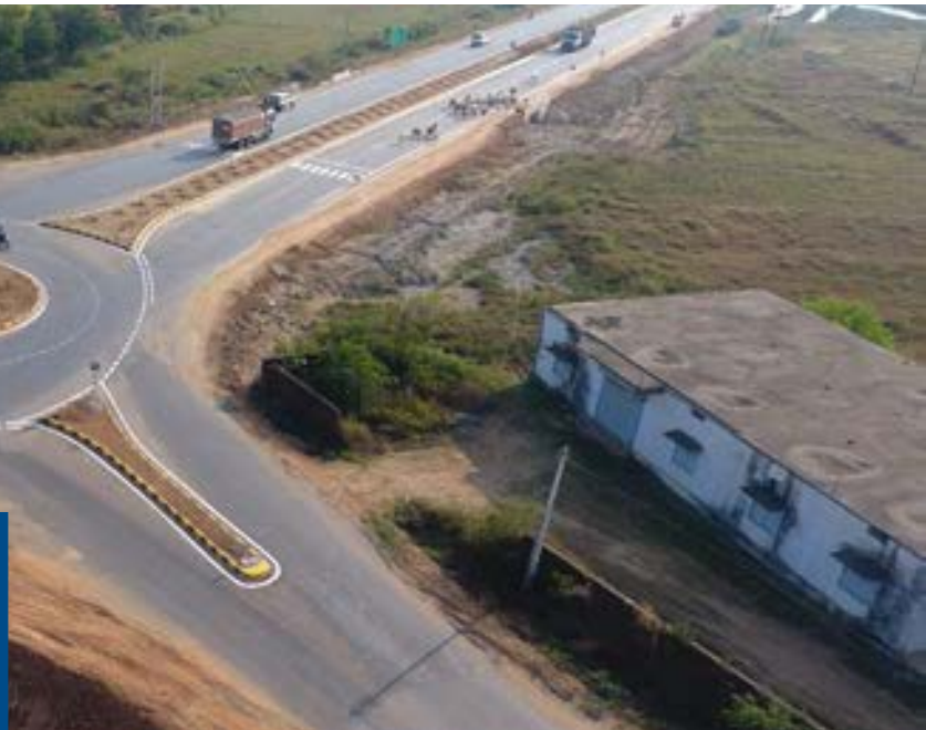
Major junction at Sambalpur-Rourkela Tollway Limited
