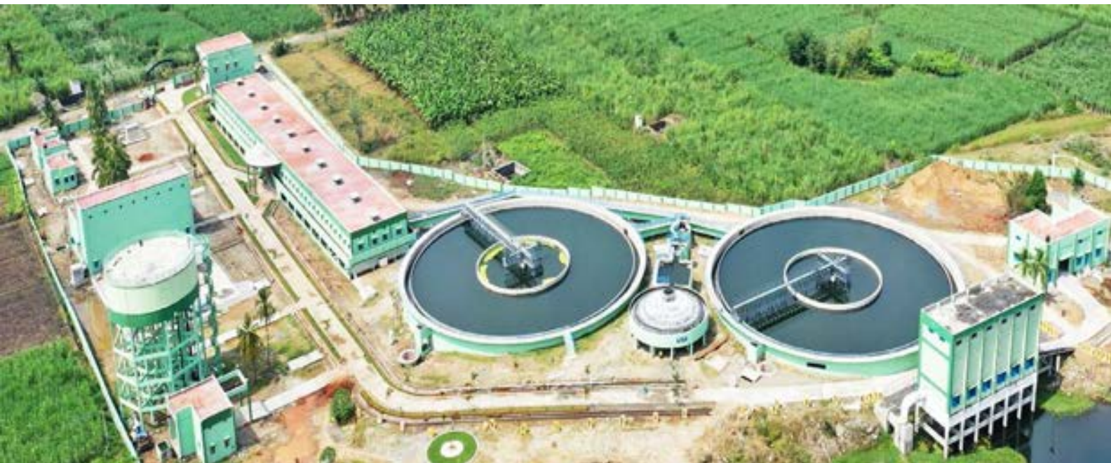
Dedicated Water Supply Project for Erode Corporation, Tamil Nadu
