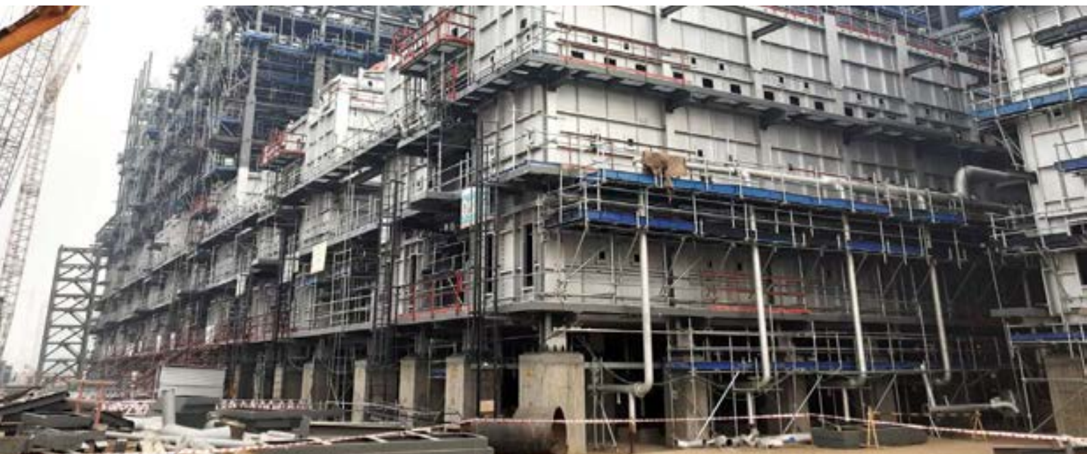
Convection modules built at MFF Hazira for HMEL Cracker Furnaces Project
