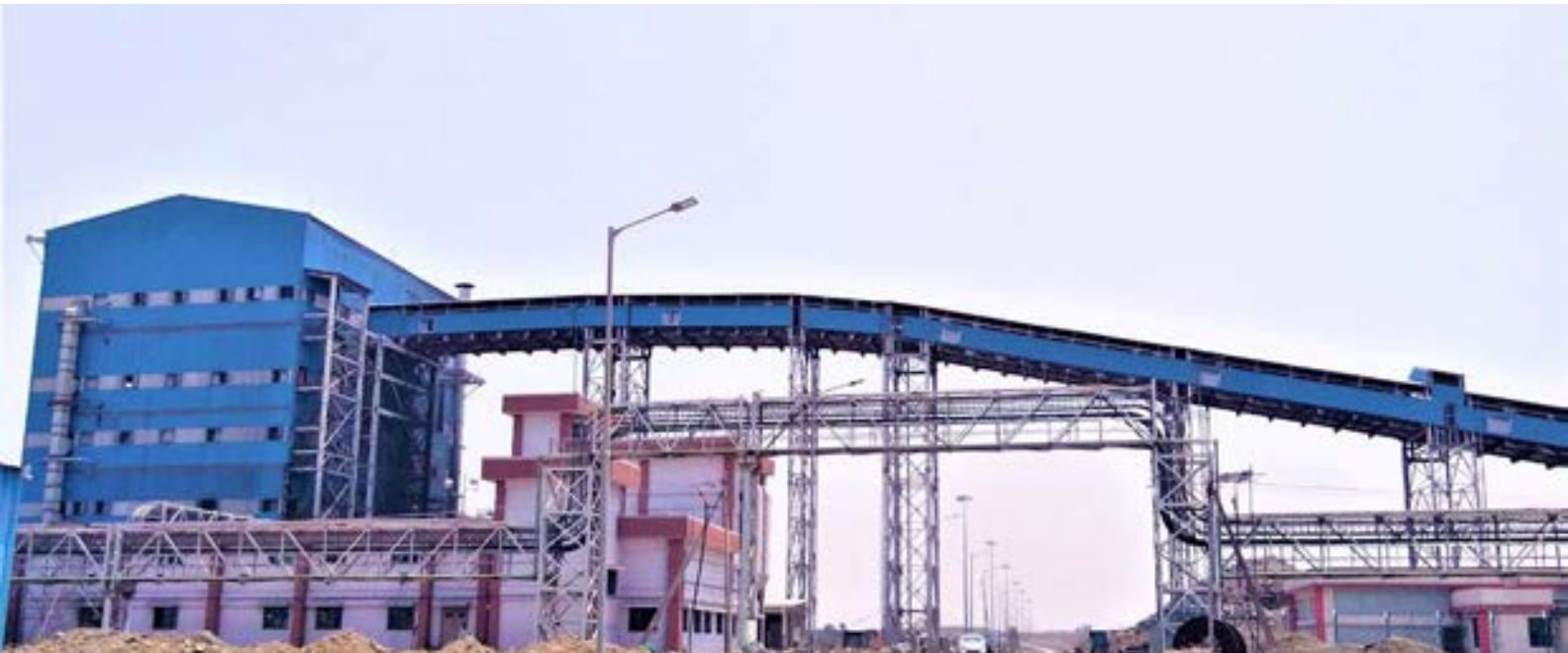
Coal-handling plant at Khargone, Madhya Pradesh
