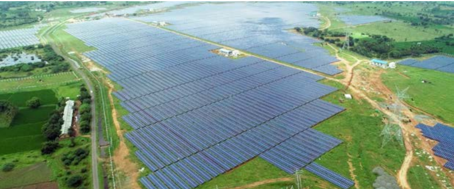
110 MWp NLC Project, Tamil Nadu
