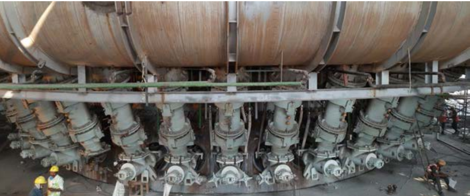
Blast furnace, JSW, Dolvi, Maharashtra
