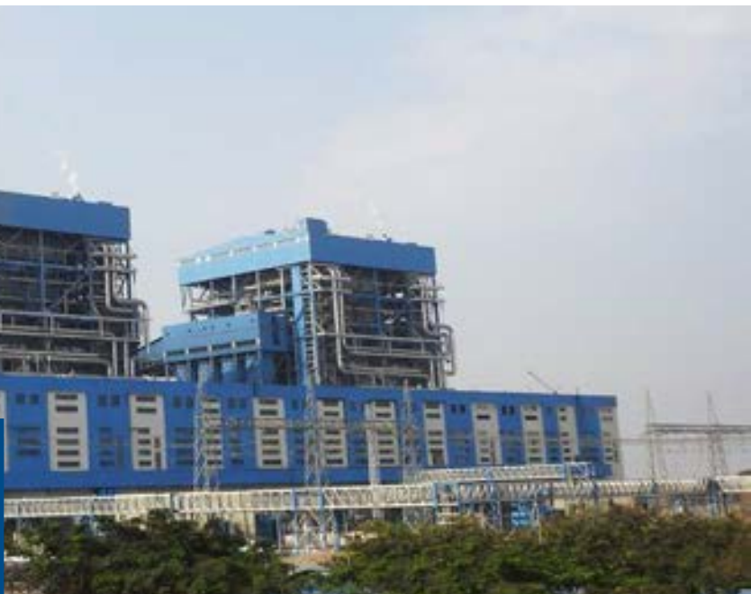
India's first ultra-supercritical power plant – 2x660 MW Khargone Thermal Power Plant, Madhya Pradesh
