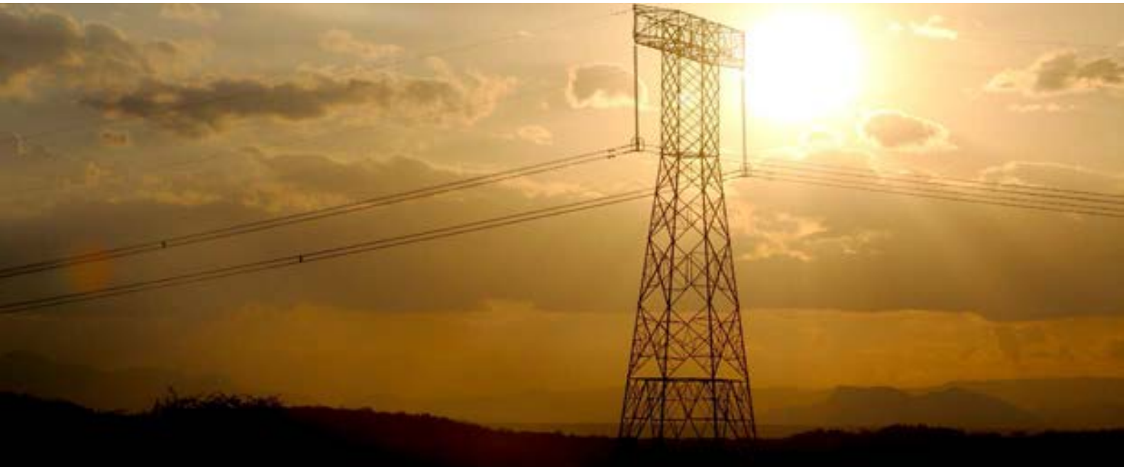
500 kV HVDC Transmission Line, Kenya
