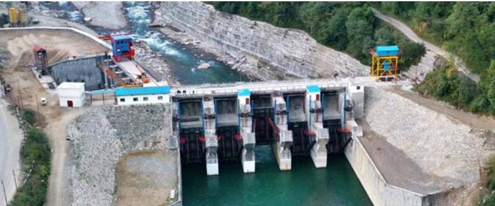
Barrage for Singoli-Bhatwari Hydro Electric Power Project (3x33 MW), Uttarakhand
