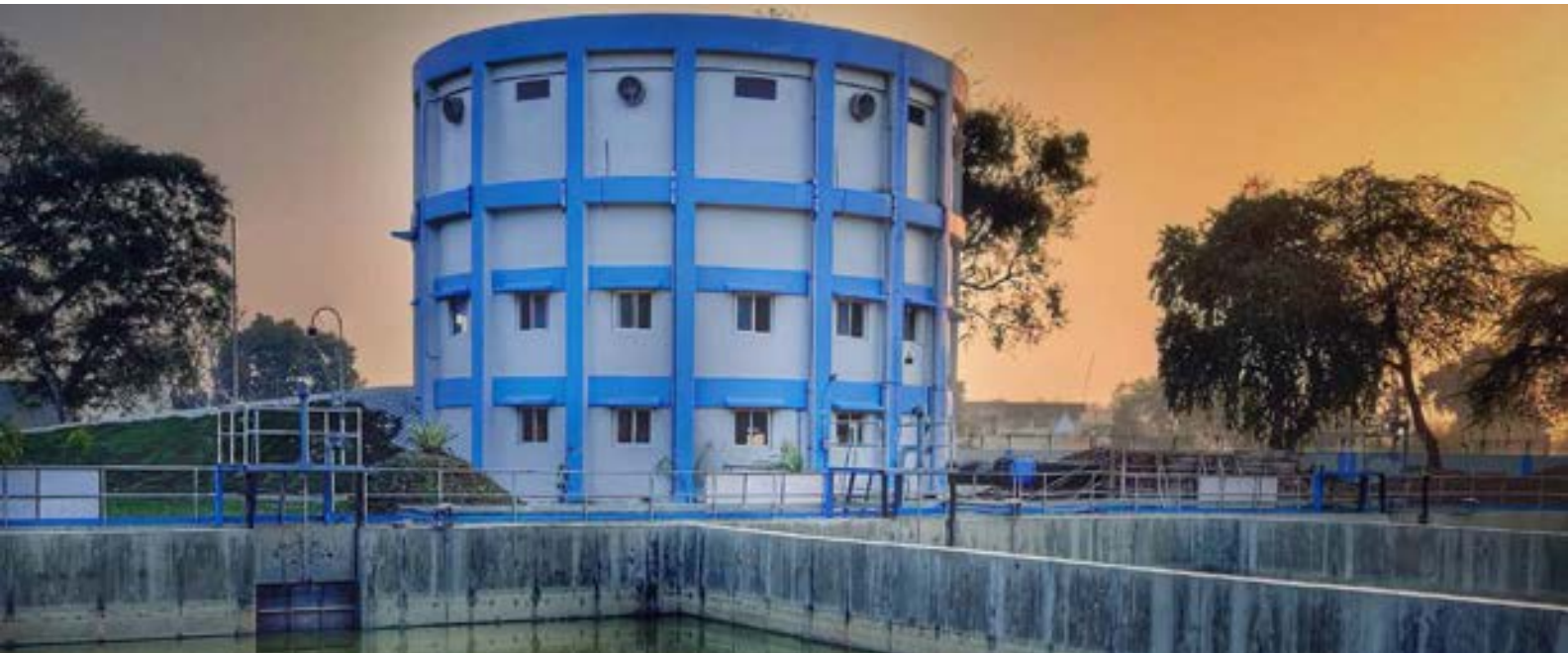
Water carrier system, Kanpur, Uttar Pradesh
