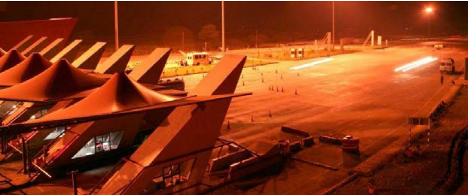
Toll plaza at Vadodara-Bharuch Tollway Limited
