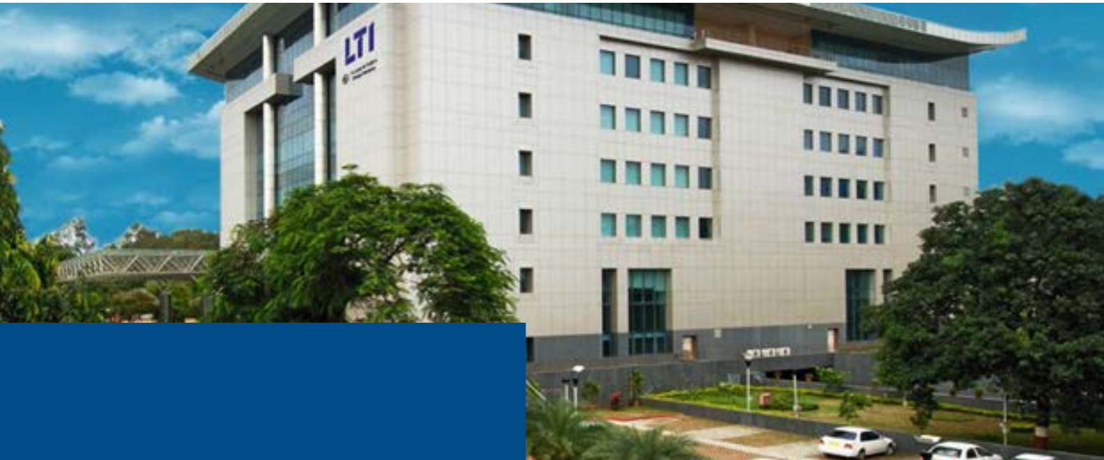
LTI Headquarters, Powai, Mumbai
