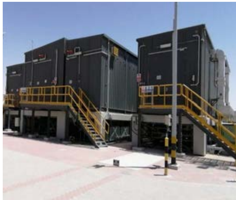
Haliba, Containerised Substation
