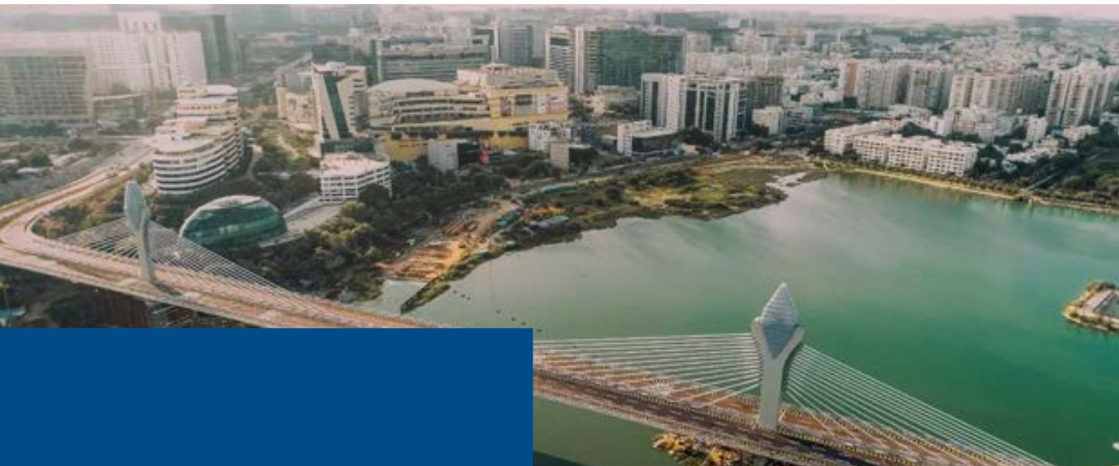
Cable-stayed bridge across Durgam Cheruvu Lake, Telangana
