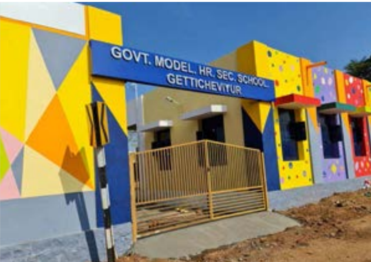
Infrastructure upgradation of a Government school at Getticheyur, Erode, Tamil Nadu
