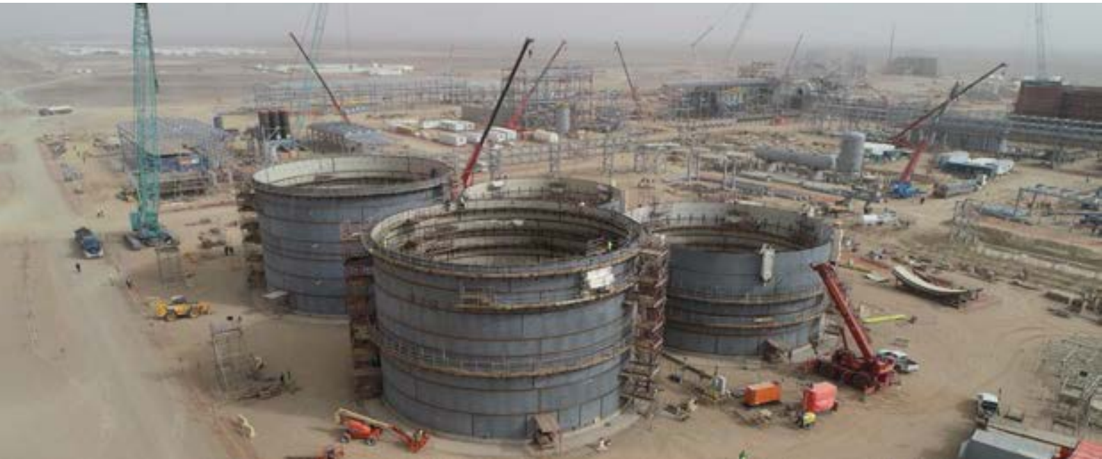
Raw Water Storage Tank for MENA, Maaden Gold Project, Kingdom of Saudi Arabia
