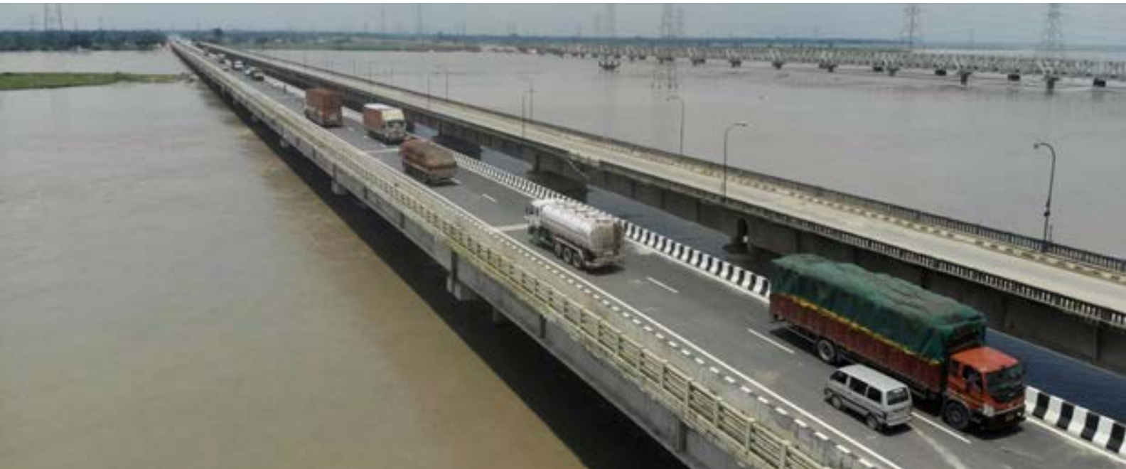
The 1-km bridge over River Teesta, Ghoshpukur-Salsalabari Road Project
