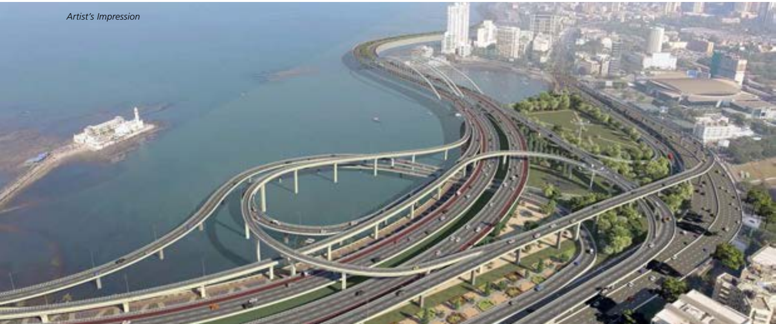
The Mumbai Coastal Road Project. L&T is executing Packages 1 and 4.
