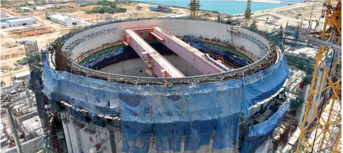
Kakrapar Atomic Power Plant 3
