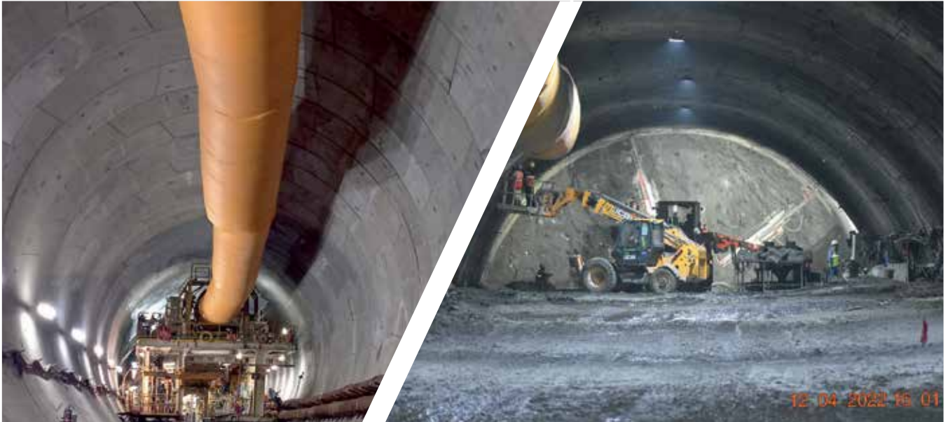
Bangalore Metro – an underground section
