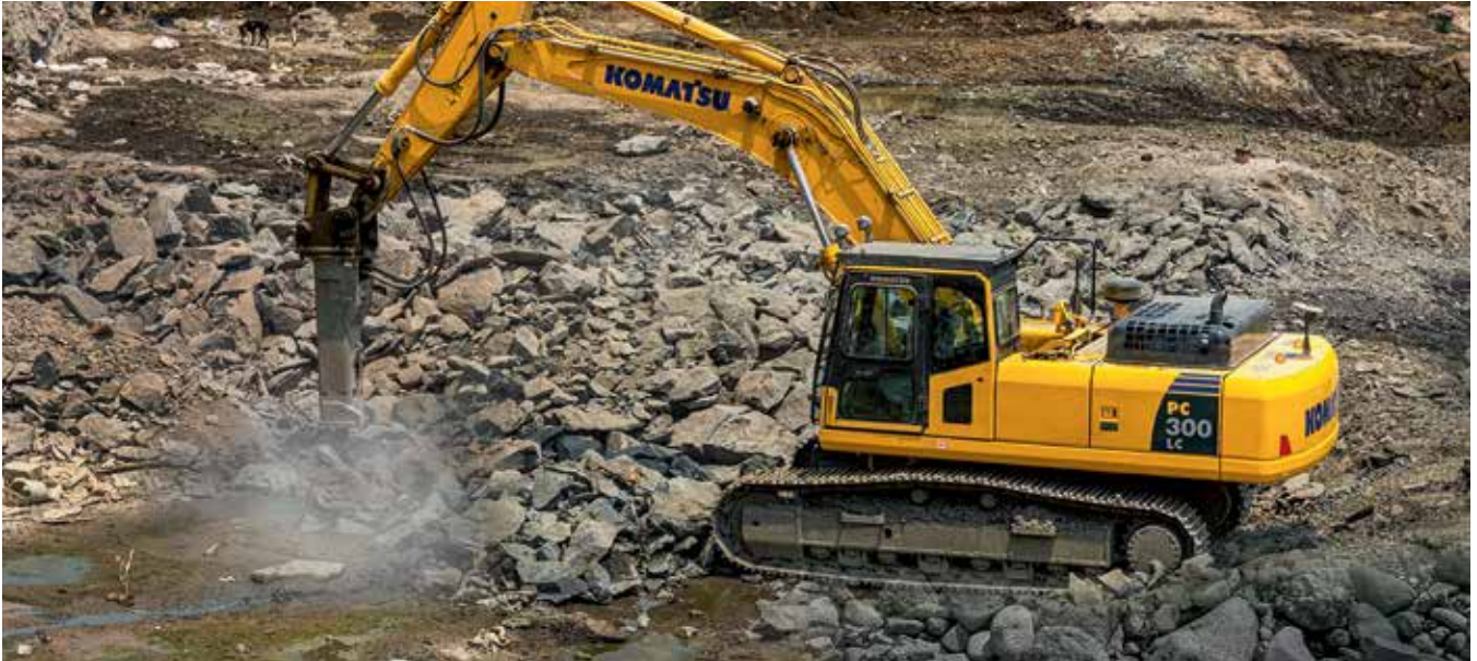
Komatsu PC300-8 Hydraulic Excavator with Breaker attachment
