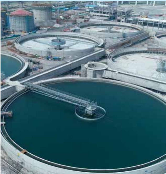
318 MLD Coronation Pillar Sewage Treatment Plant, Delhi
