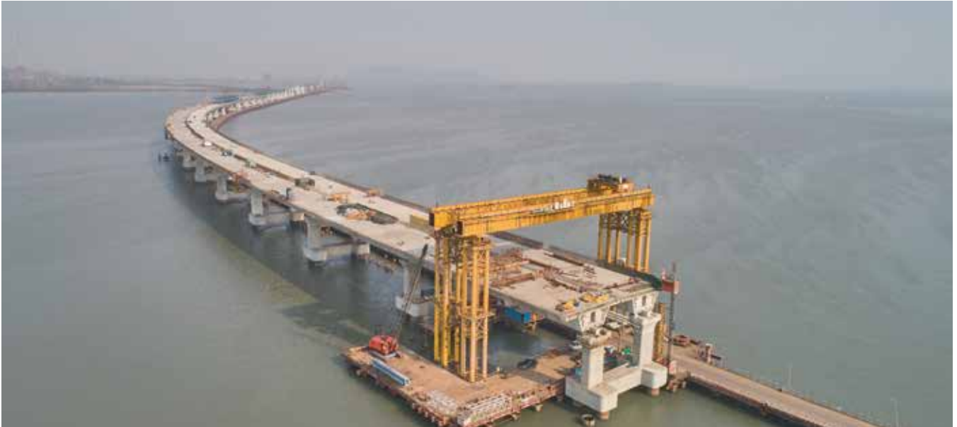
Mumbai Trans Harbour Link Project
