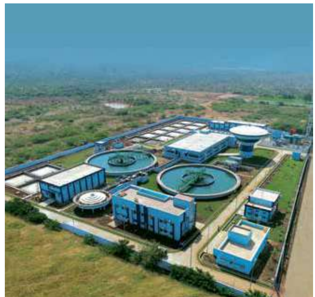
48 MLD Water Treatment Plant, Gadag, Karanataka
