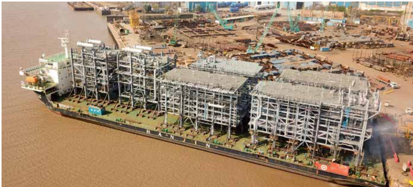
Onshore Process & Piperack Modules being loaded-out from MFF Hazira for a Refinery in Thailand
