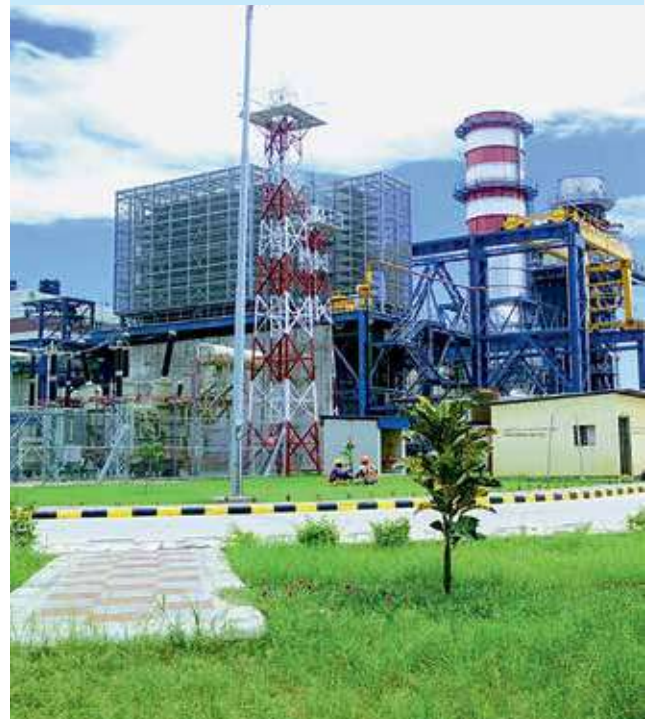
400 MW Bibiyana-III Combined Cycle Power Plant, Bangladesh
