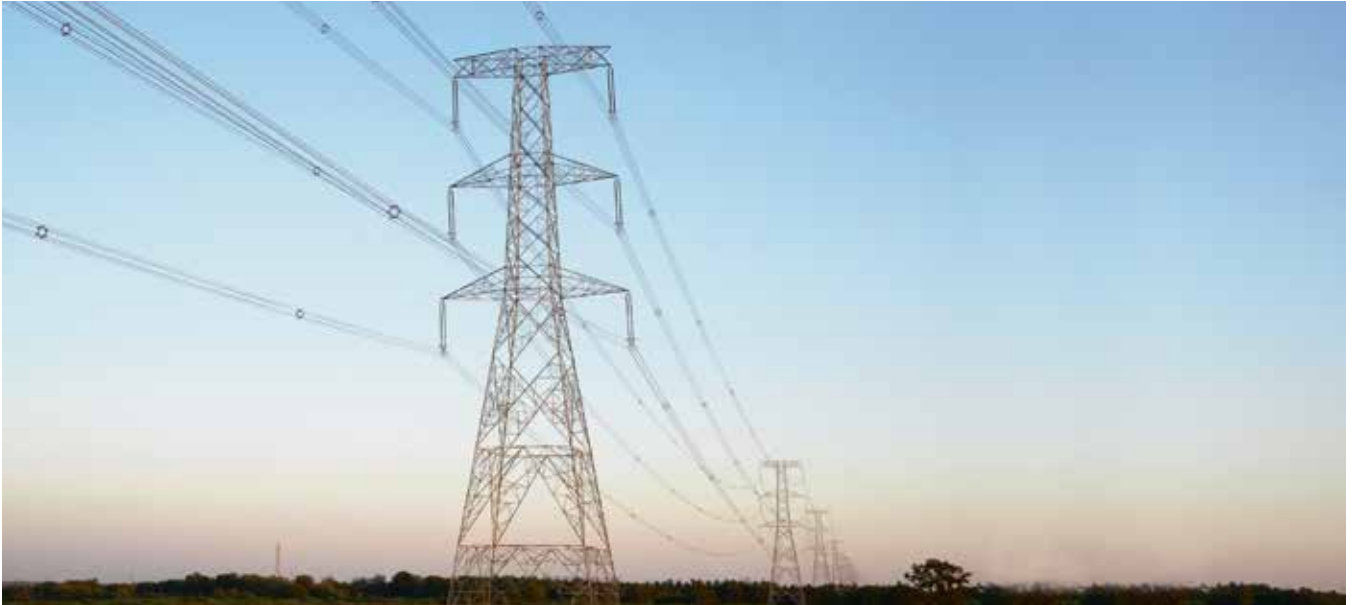
Kudgi Transmission Lines, Karnataka
