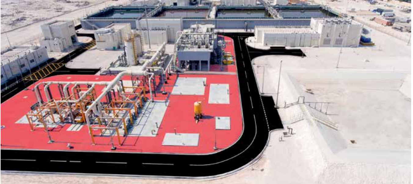
Industrial Area Sewage Treatment Works, Doha, Qatar
