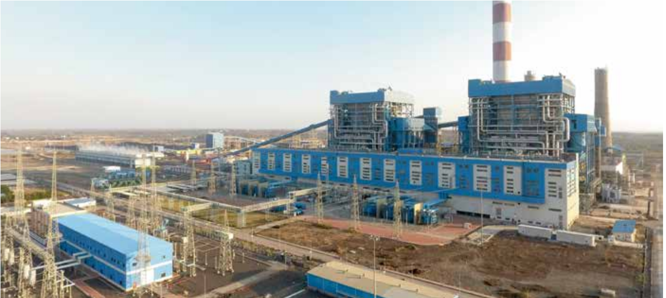
2x660 MW Khargone Thermal Power Plant, Madhya Pradesh (India's first ultra-supercritical power plant)
