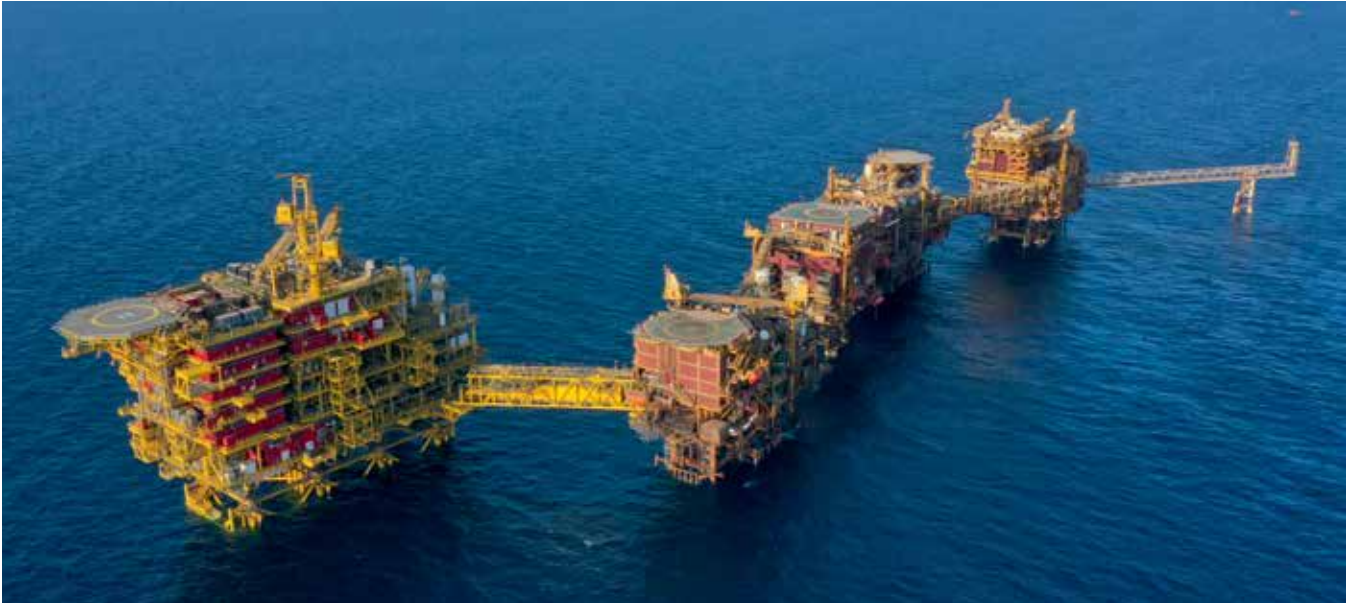
New Water Injection South - R Project for ONGC
