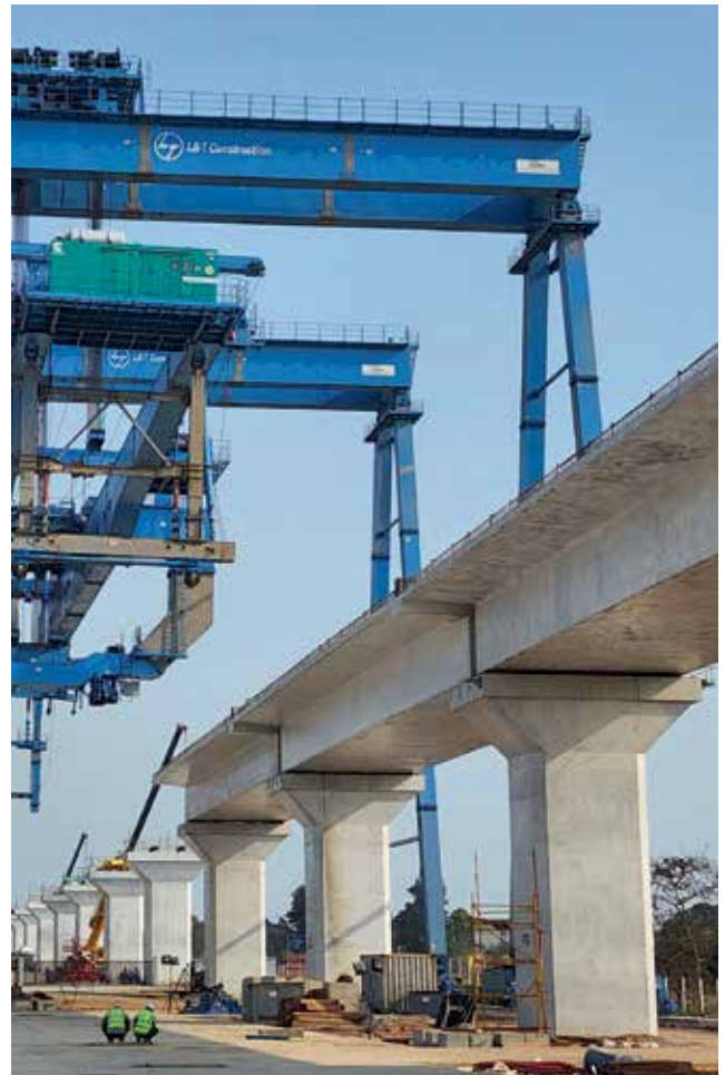
Mumbai - Ahmedabad High-Speed Rail Project
