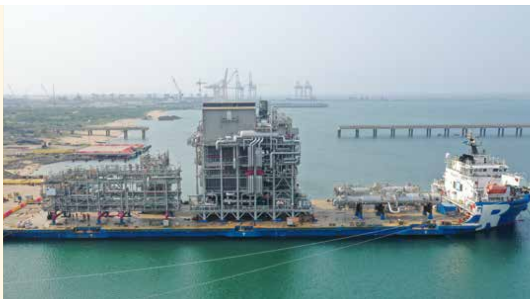
Modularised Reformer for a Blue Hydrogen project in Rotterdam, Netherlands
