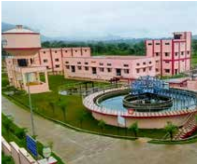
Water Treatment Plant
