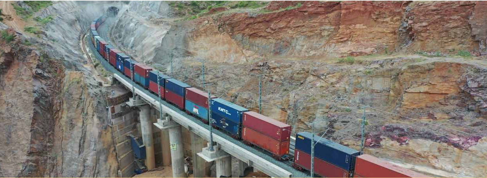
Western Dedicated Freight Corridor (Civil & Track Package 14), Haryana-Uttar Pradesh
