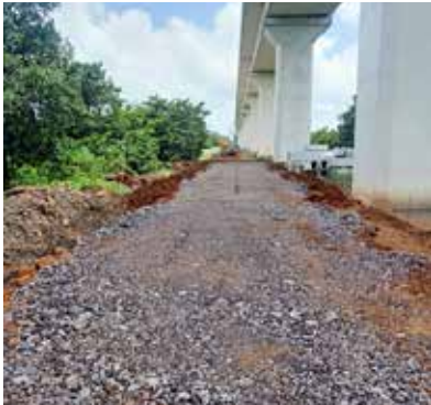
Approach road using steel slag
